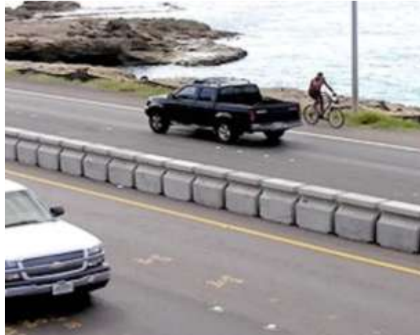
Figure 5-110: Concrete Reactive Tension System Barrier Photo Courtesy of Lindsay Transportation
