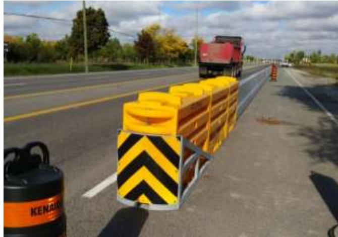
Figure 5-285: SLED Temporary Reduced Exposure Energy Attenuator
