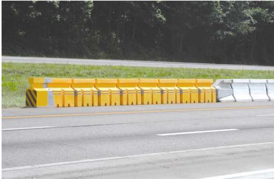
Figure 5-252: Absorb 350 Temporary Reduced Exposure Energy Attenuator
