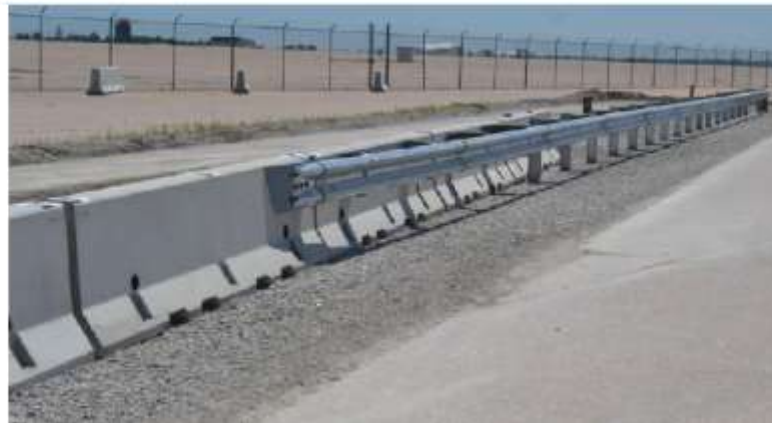
Figure 5-296: Transition from Existing SBGR to TCB Photo courtesy of MwRSF
