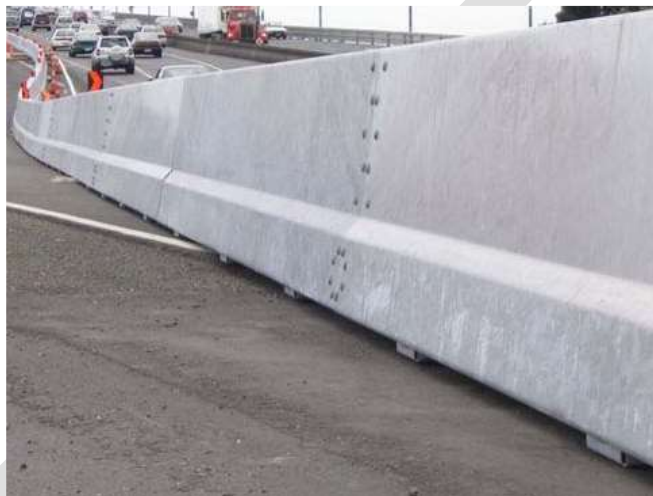
Figure 5-174: BarrierGuard 800 Temporary Steel Barrier
