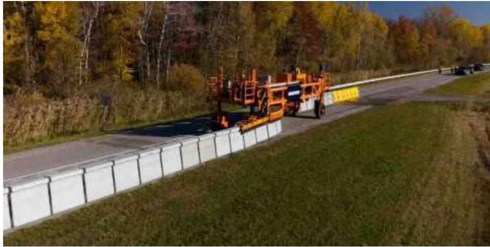
Figure 5-15XX: TALL42 Moveable Barrier Transfer Machine Shifting Barriers
