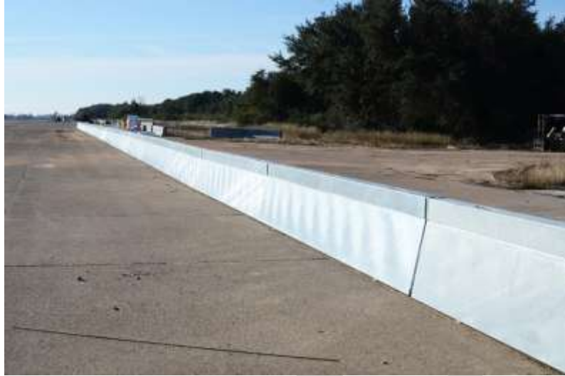
Figure 5-2148: HV2 Temporary Steel Barrier Photo Courtesy of Safe Roads
