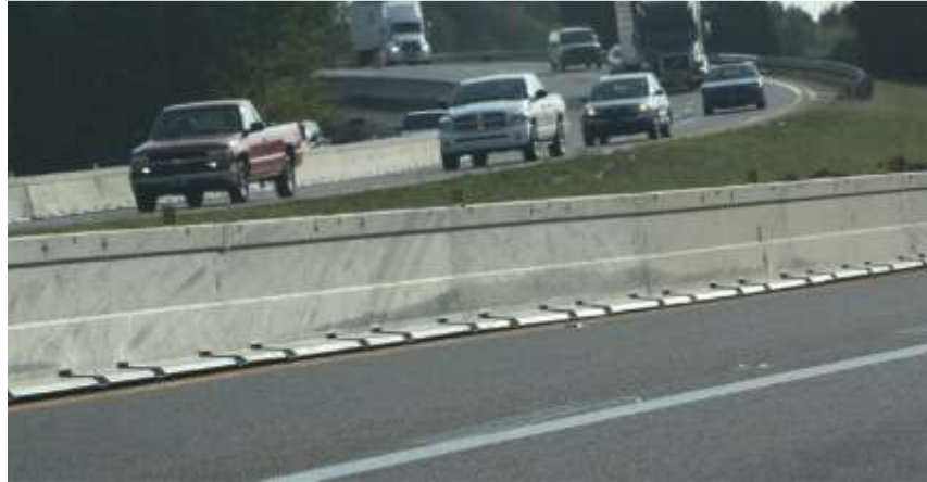
Figure 5-158: ZoneGuard Temporary Steel Barrier Installation
