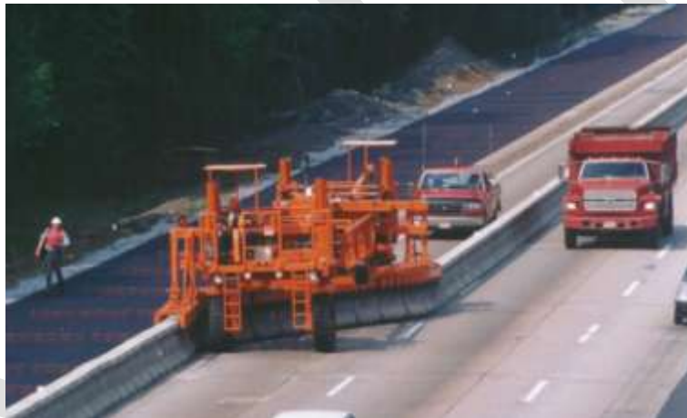
Figure 5- 98 : Quickchange Moveable Barrier Transfer Machine Shifting QMB Barrier
