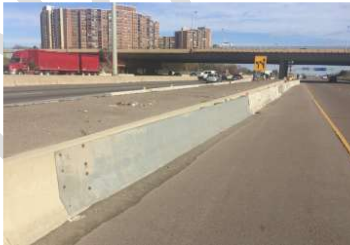
Figure 5-3027: Transition from Permanent Concrete Barrier to Temporary Concrete Barrier Photo courtesy of Powell Construction and TTI.
