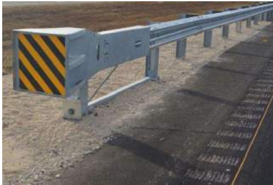
Figure 4-350: MSKT Installation
