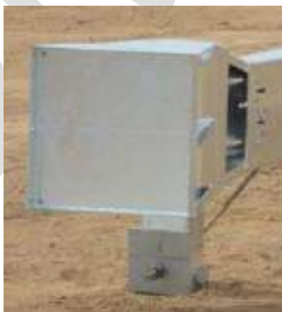
Figure 4-3634: Correct Orientation of Bearing Plate on Compression Based Terminals Photo courtesy of Road Systems, Inc.
