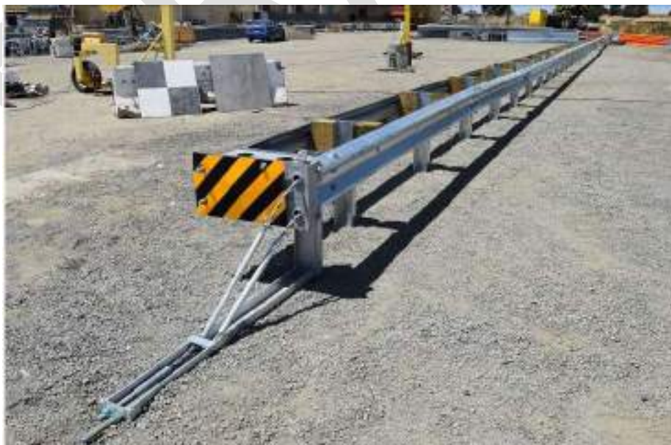
Figure 4-4033: Max Tension Median Terminal Installation
