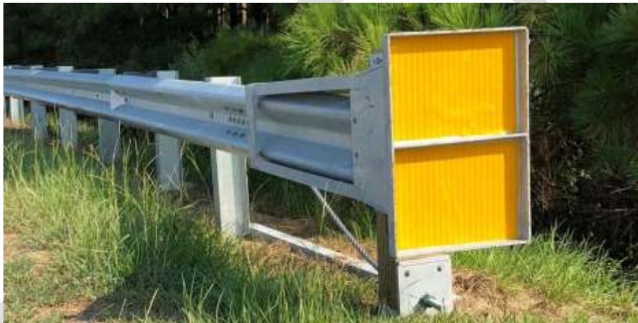
Figure 4-372: SPIG Gating End Terminal Installation Photo courtesy of SPIG Industries
