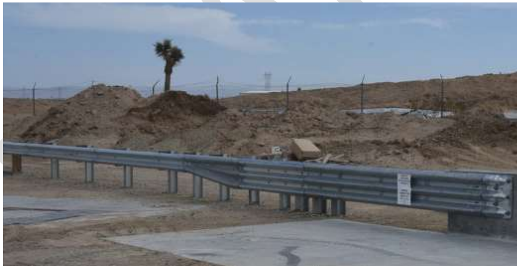
Figure 4-141: Legacy SBGR with Channel Connection to Concrete Parapet Wall, See applicable standard drawing for Notes
