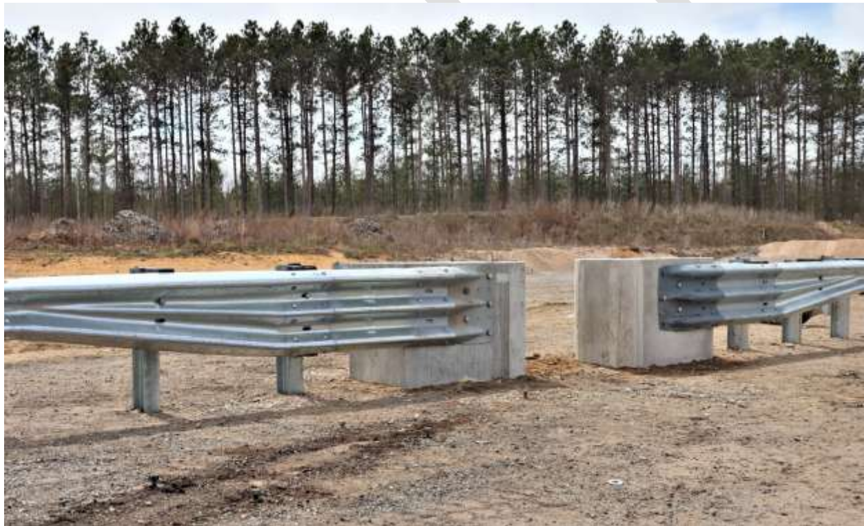
Figure 4-130: Pedestrian Access Terminal (PAT) for Steel Beam Guide Rail, courtesy of Northern Infrastructure Products ( www.northern-ip.com )
