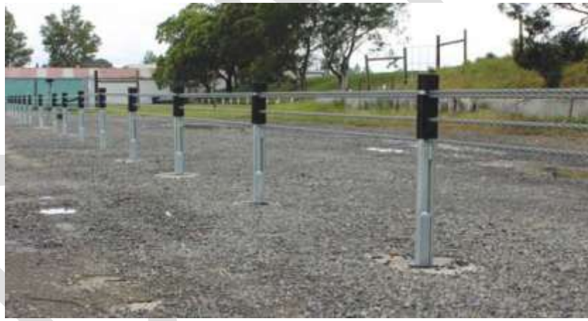
Figure 4-32: Safence HT4CGR Installation
