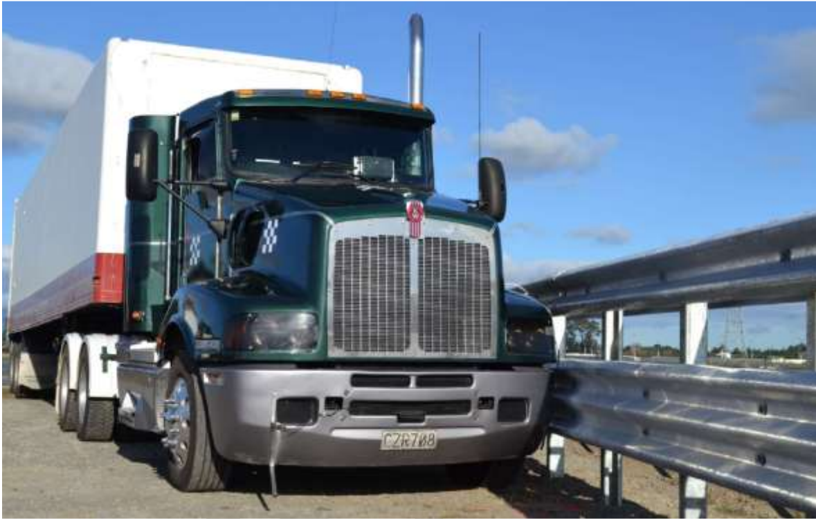
Figure 4-3025: Guardian 5 Steel Beam Median Barrier System
