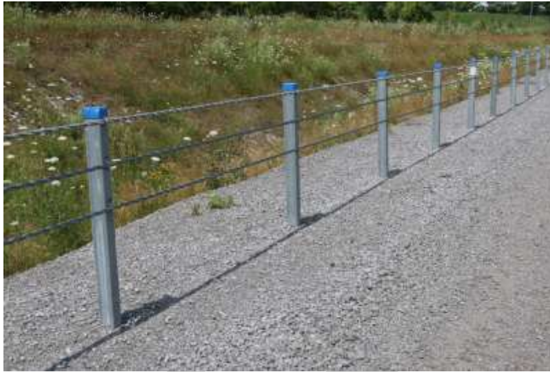
Figure 4-21: Safence HT3CGR Installation
