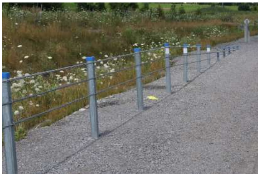
Figure 4-42: Safence HTCGR installation
