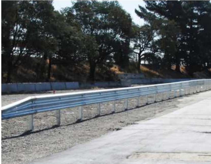
Figure 4-2519: ACP TL-4 Barrier
