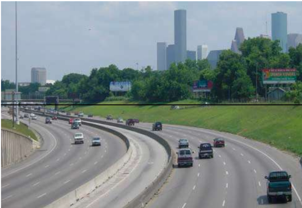
Figure 12.11.3 Freeway Median Busway (Interstate 45, Huston, Texas)
