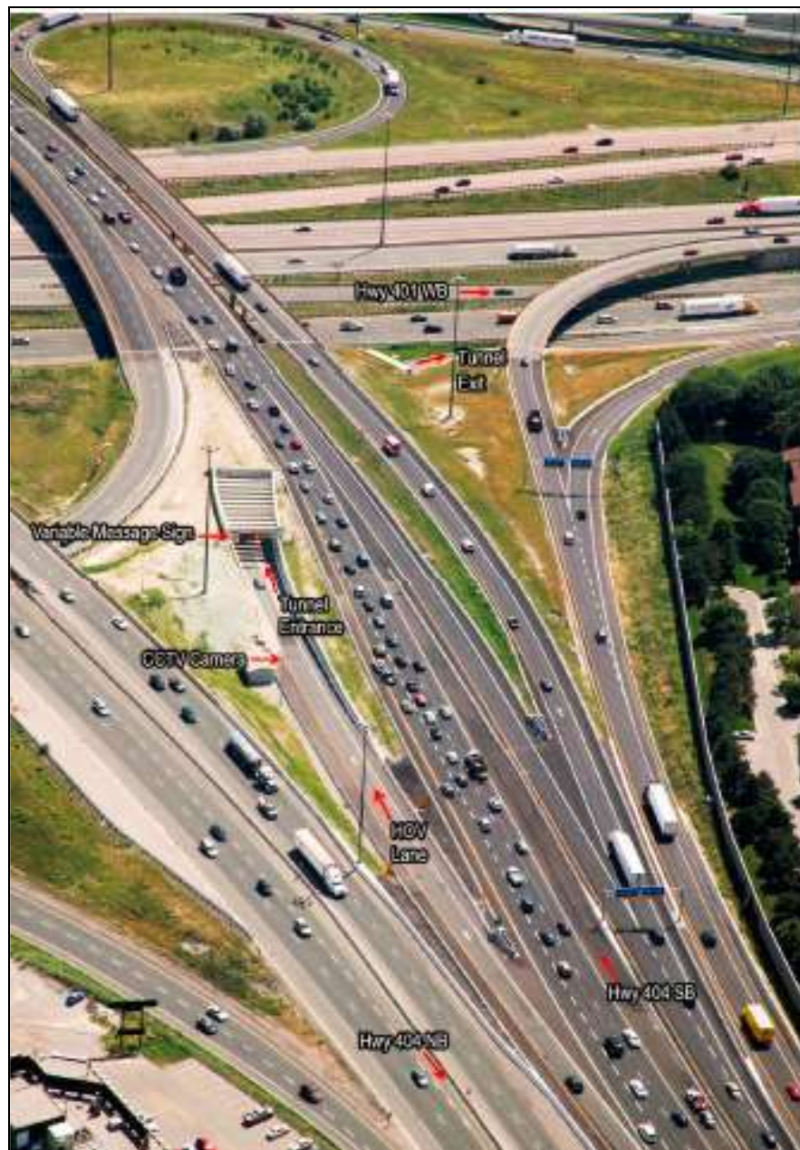
Figure 12.7.3 Highway 404 and Highway 401 VMS at Tunnel Entrance
