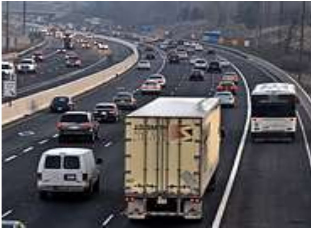
Figure 12.11.14 Bus ByPass Shoulders
