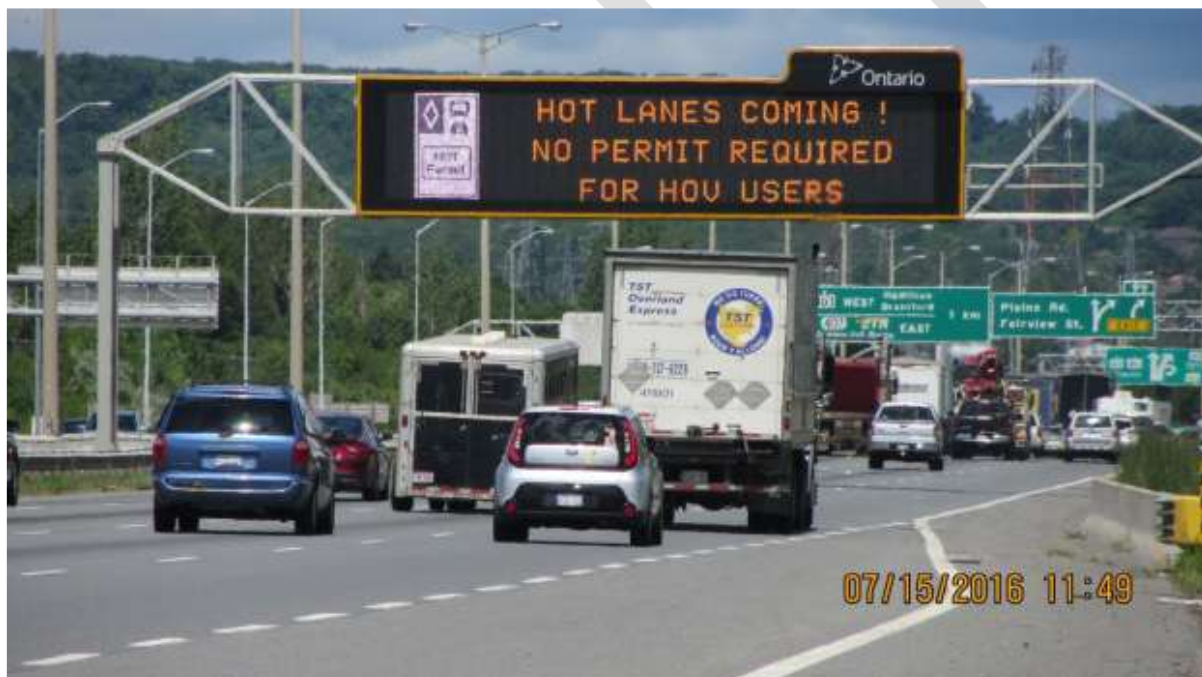
Figure 12.1.2 HOT Lanes Pilot Digital Message Signs
