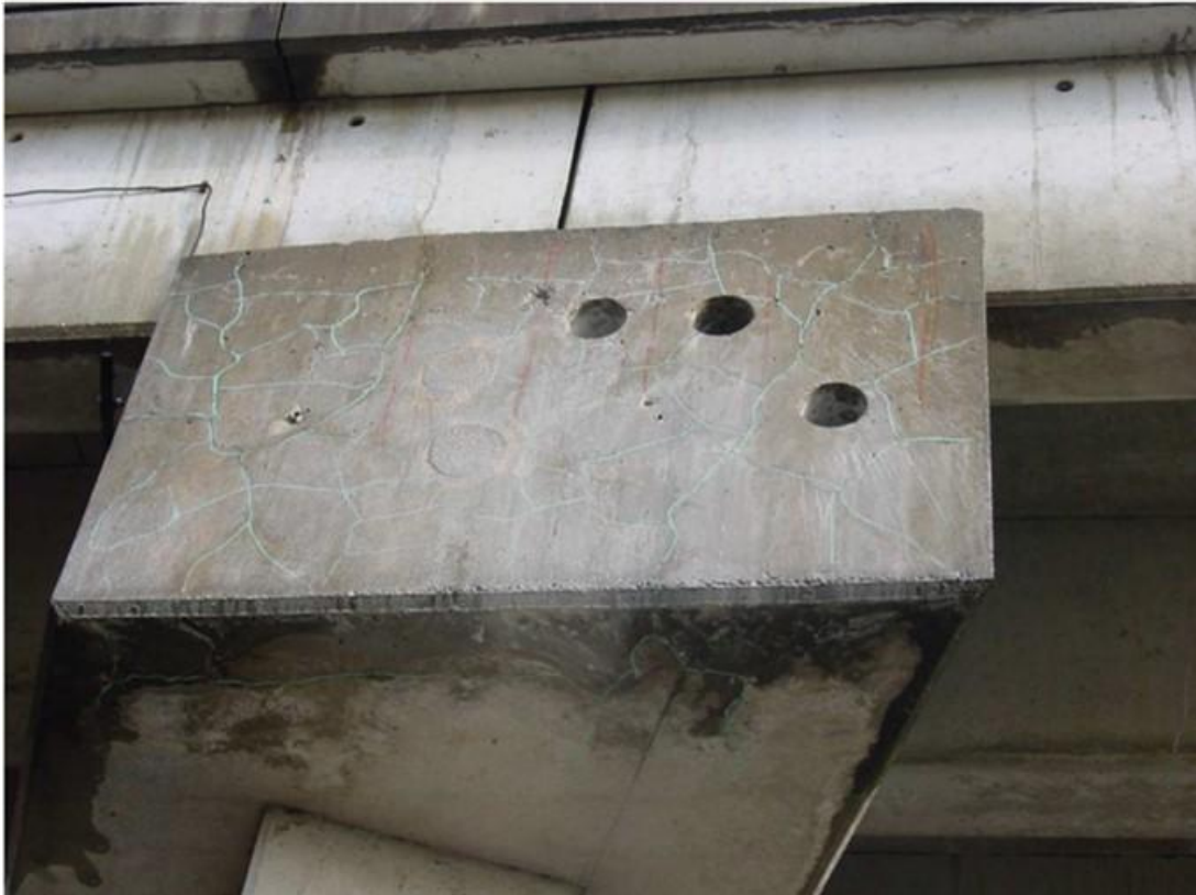
Figure A.12 (g) – Pier Cap
