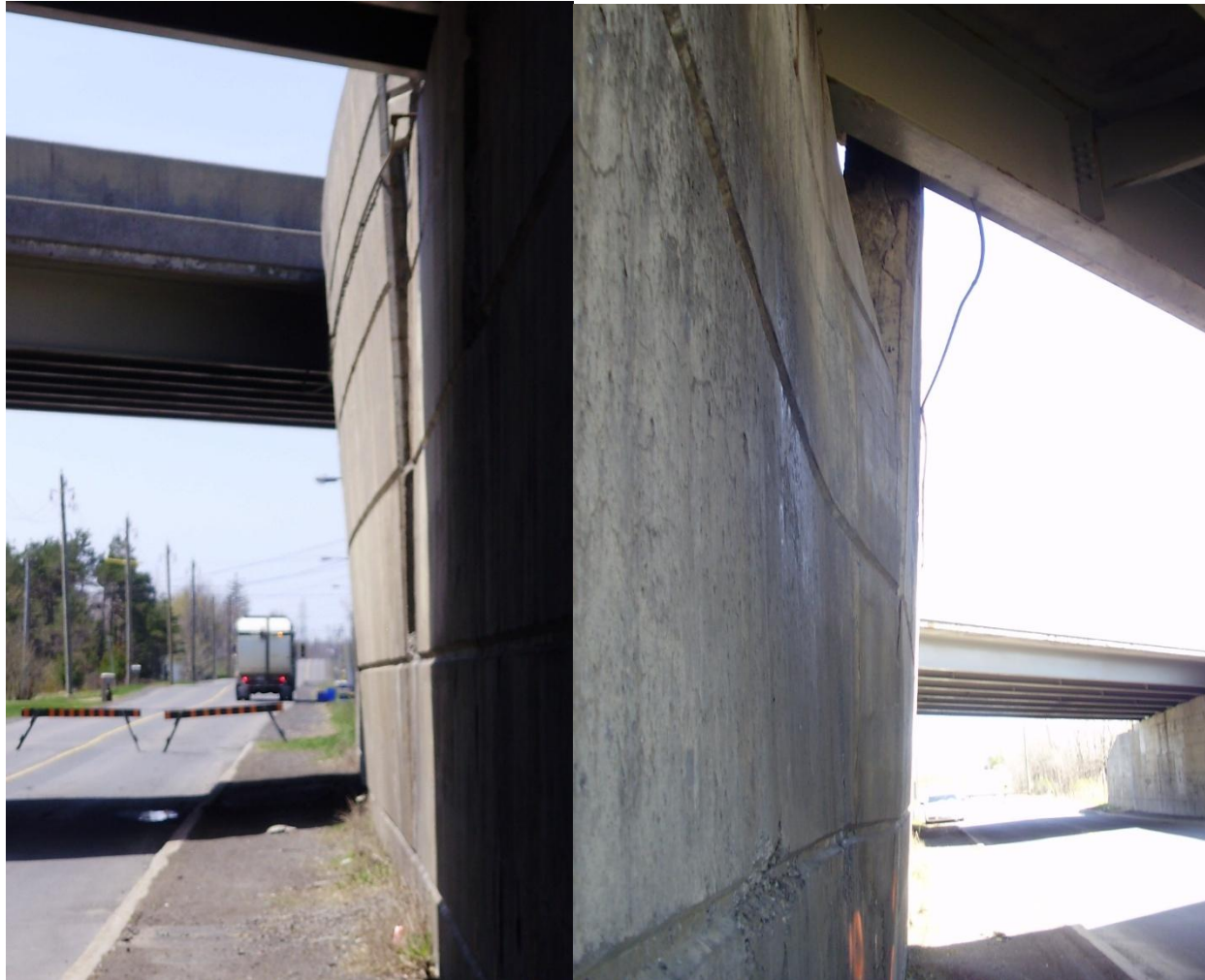
Figure A.13 (c) Cast-in-place Retaining Wall
