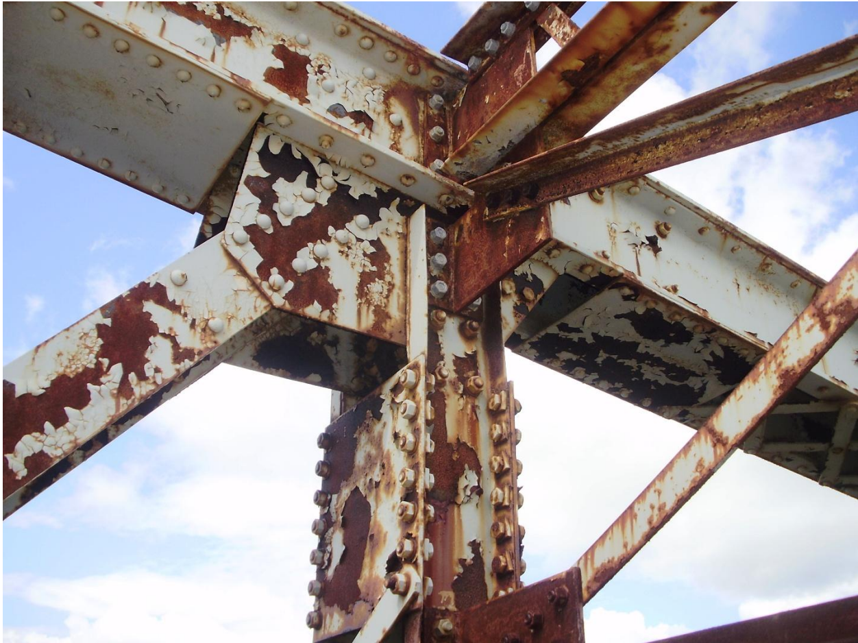
Figure A.14 (a) Steel Through Truss Connection
