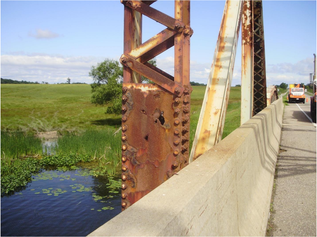
Figure A.14 (c) Vertical Member of Steel Through Truss
