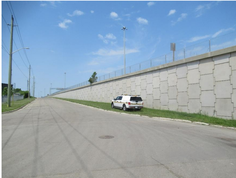
Figure A.13 (a) Precast Concrete Retaining Wall
