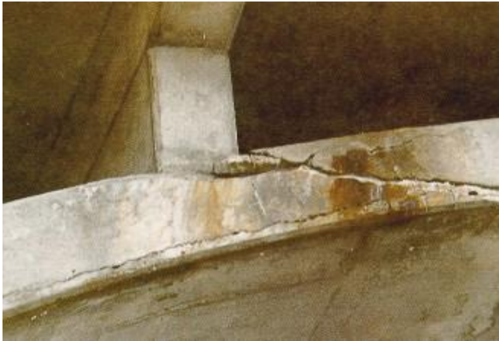
Figure A.14 (e) Concrete Spandrel Arch
