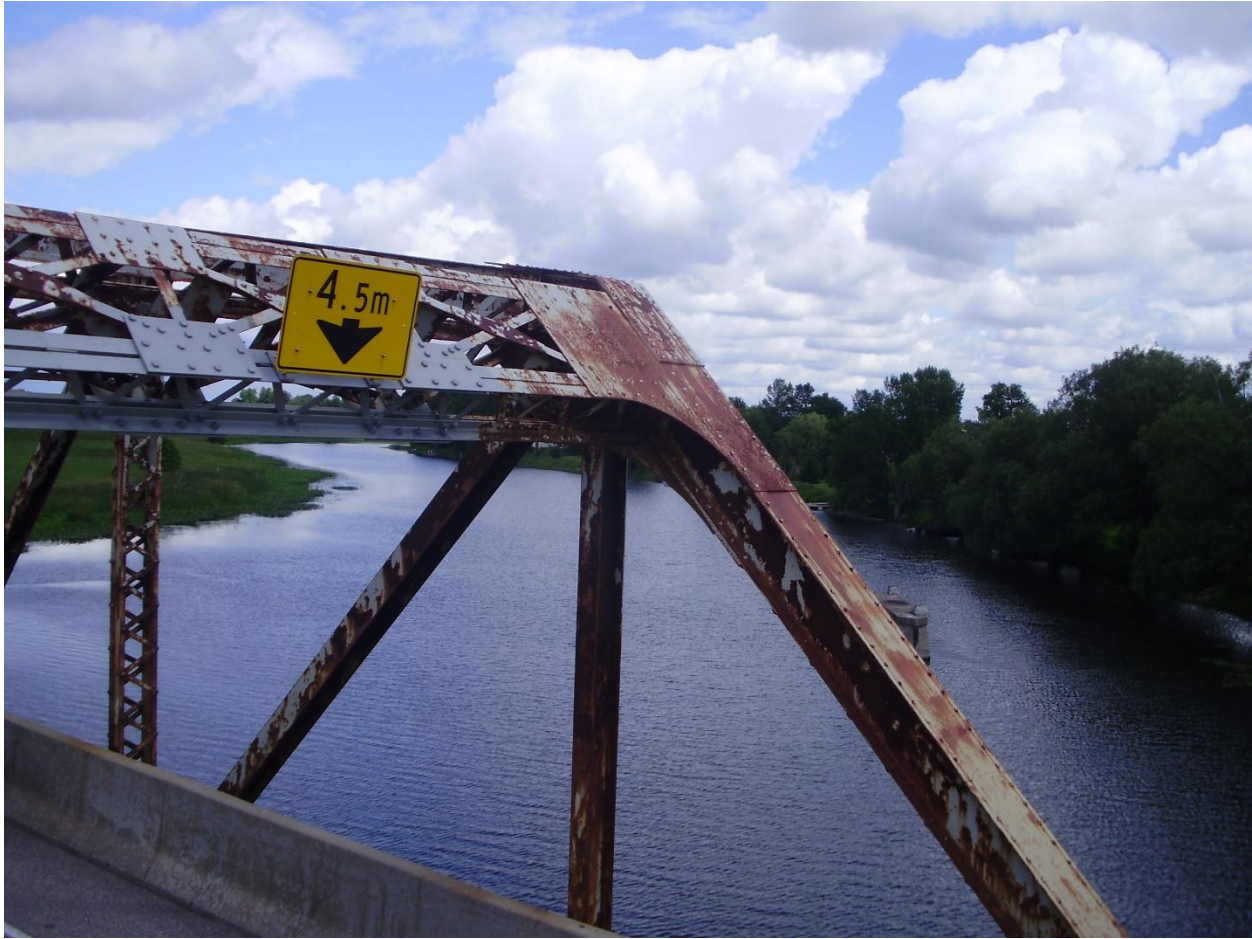
Figure A.14 (b) Sway Frame Connection
