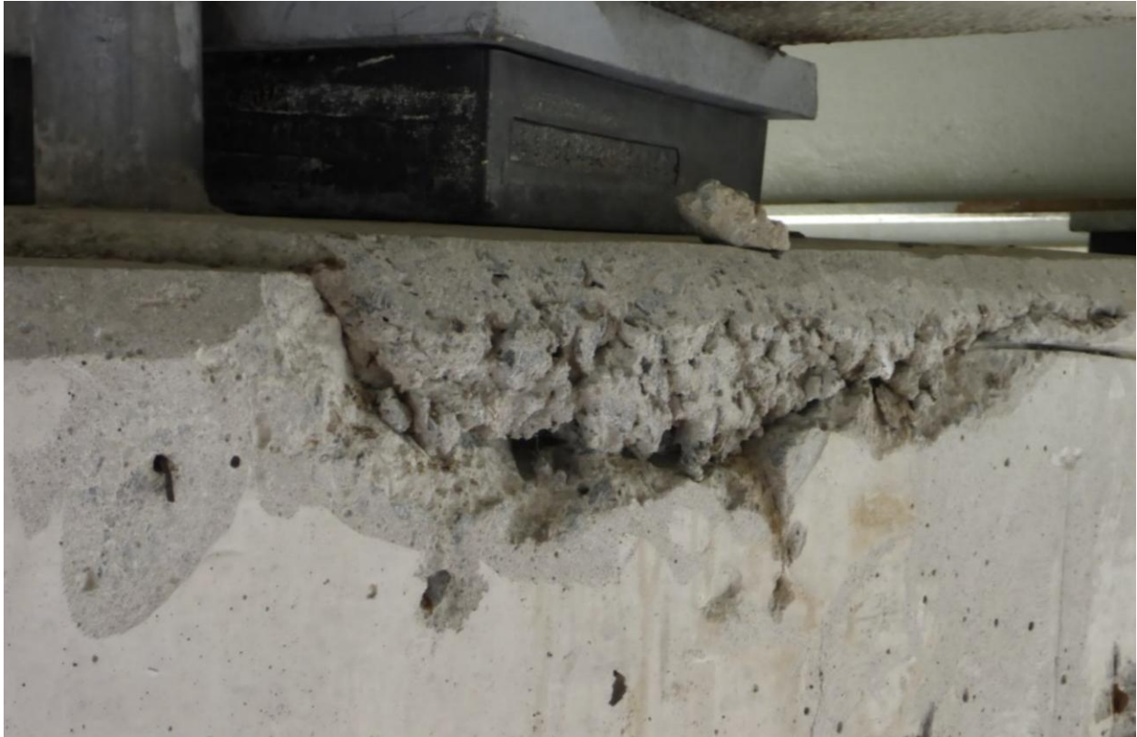
Figure A.12 (f) Concrete Pier Cap
