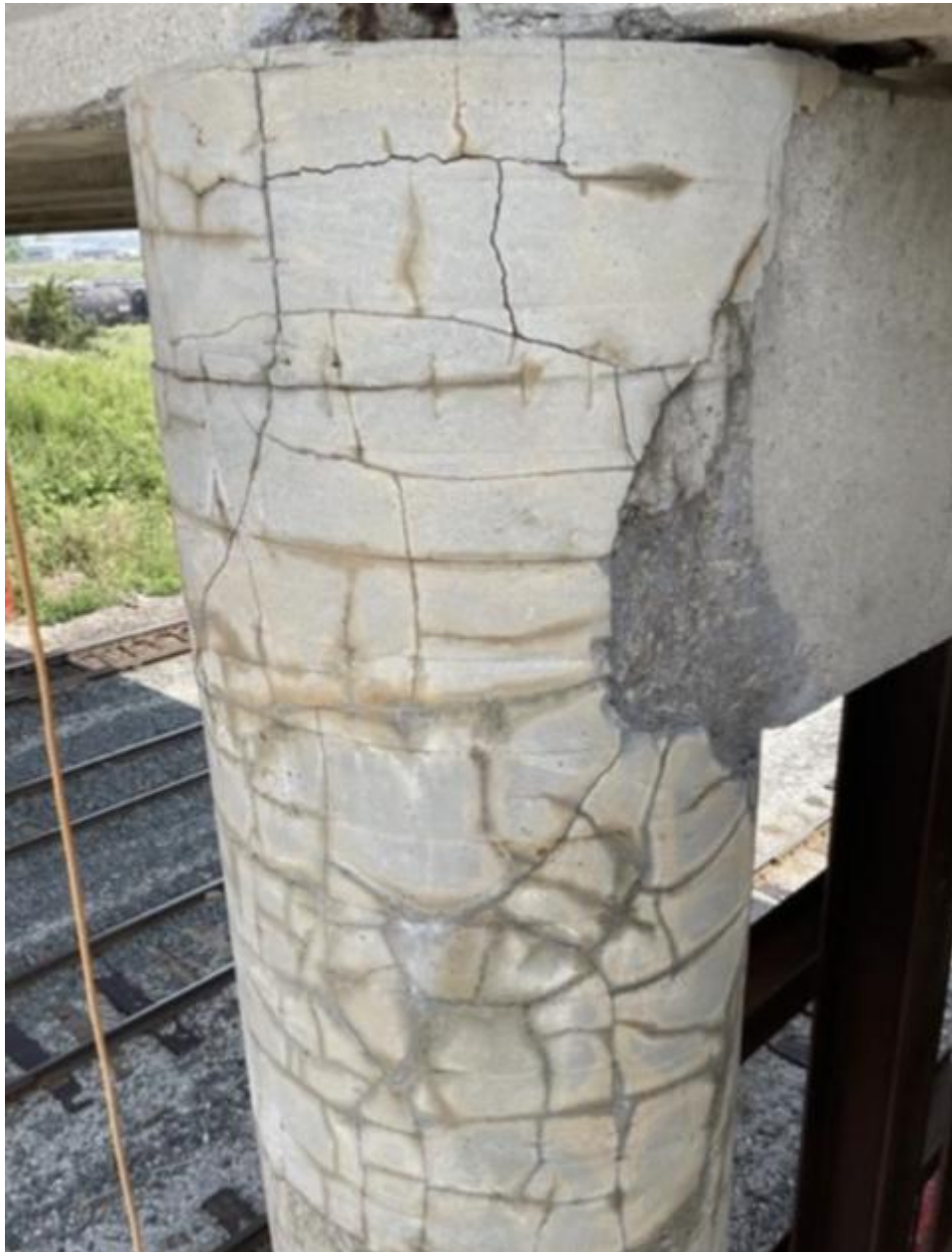
Figure A.12 (b) Concrete Pier Column
