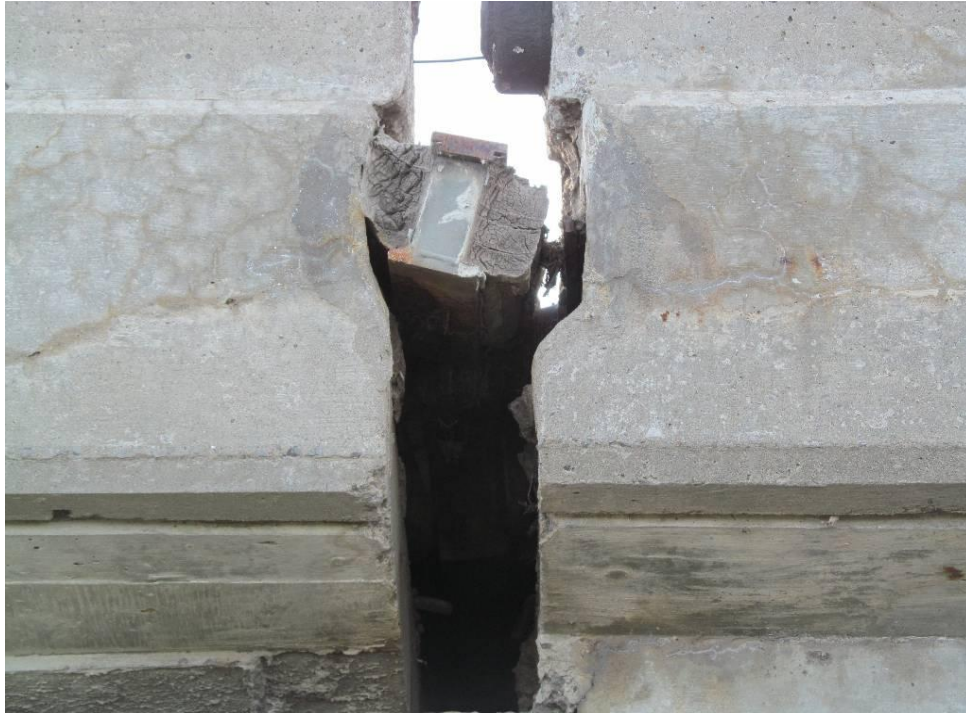
Figure A.11 (b) Compression Seal Joint
