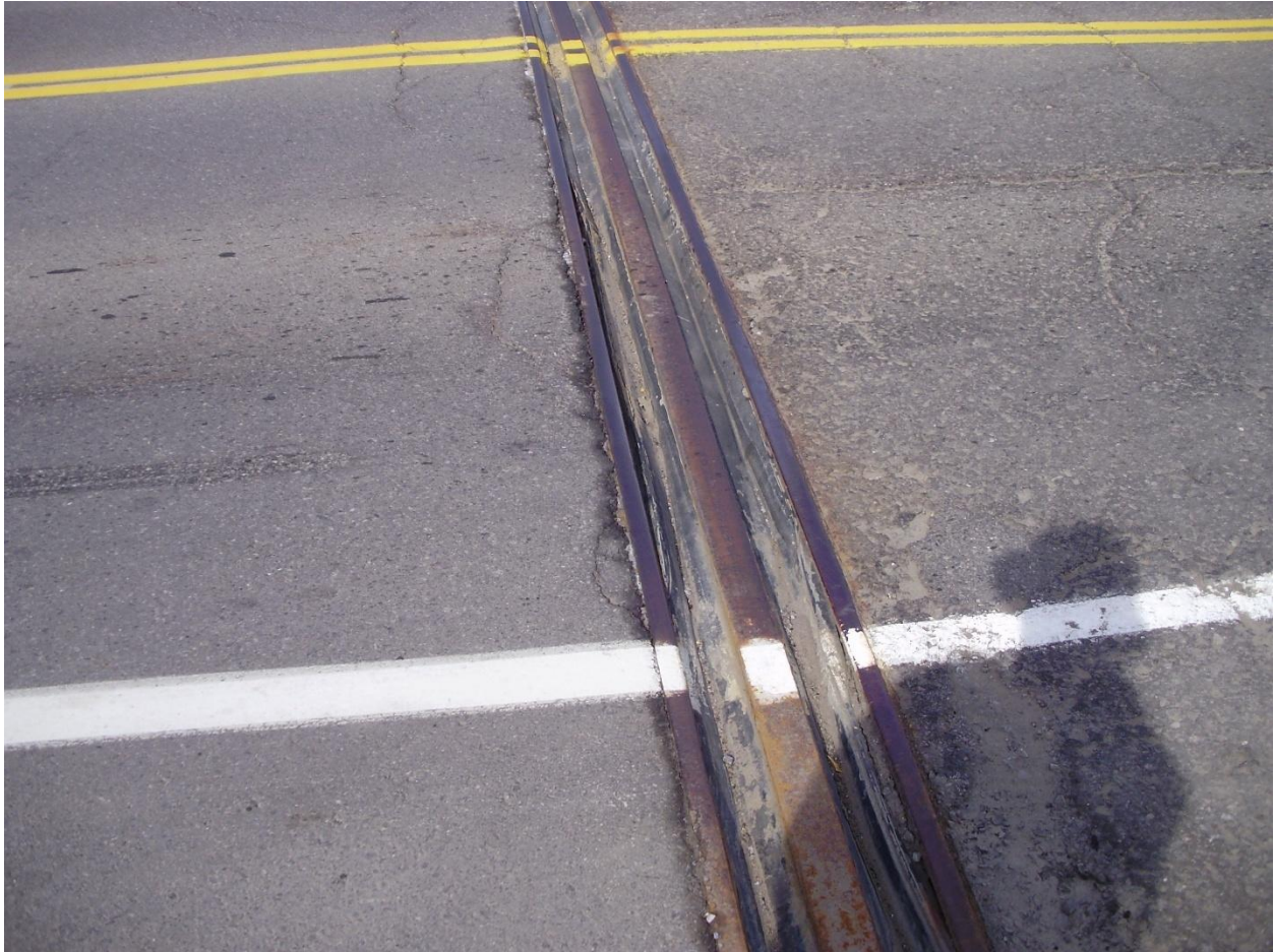
Figure A.11 (e) Multiple Seal Joint
