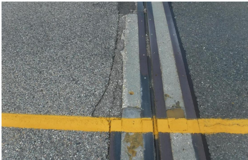
Figure A.11 (g) Expansion Joint Armouring
