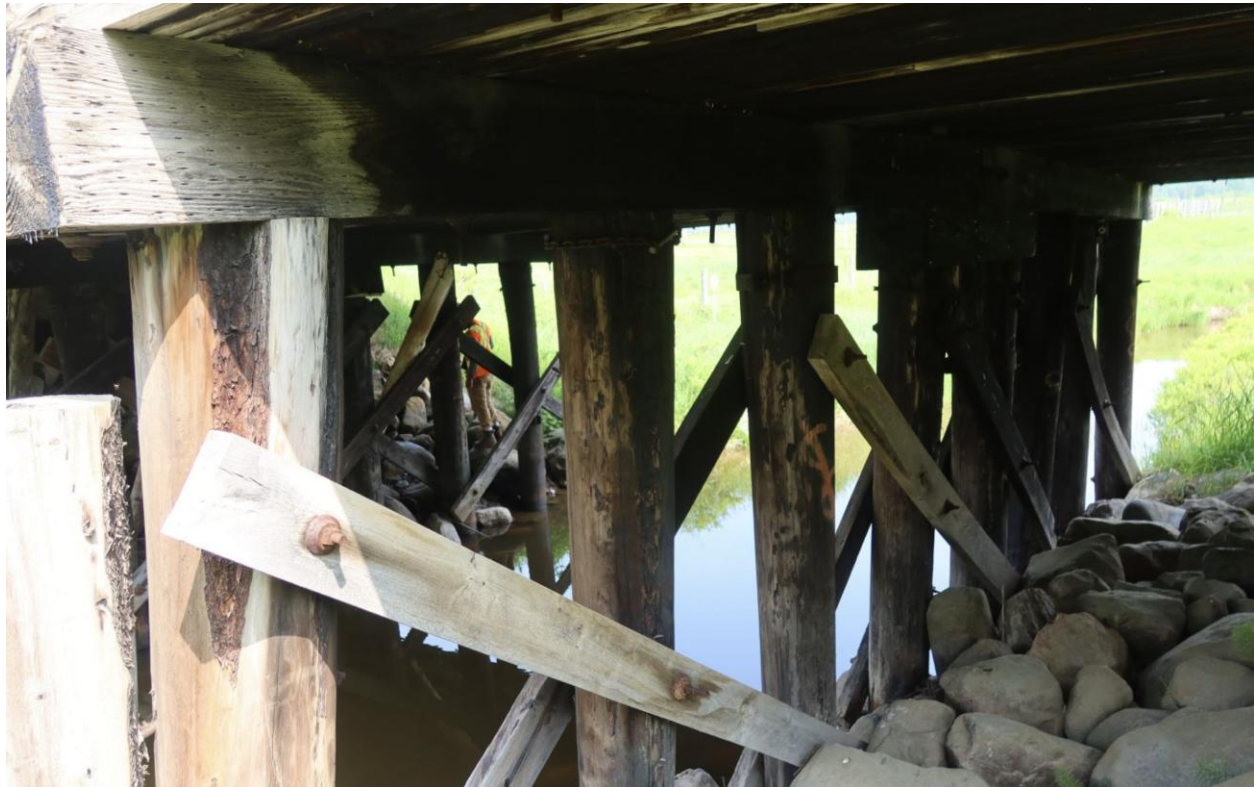
Figure A.12 (c) Wood Pier Columns
