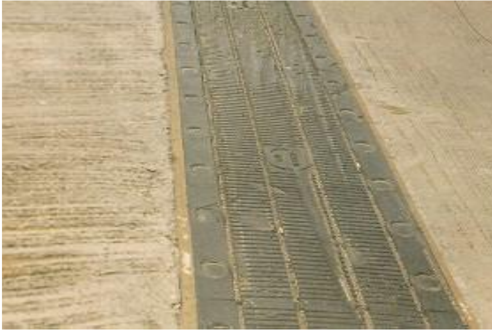
Figure A.11 (f) Rubber Cushion Joint
