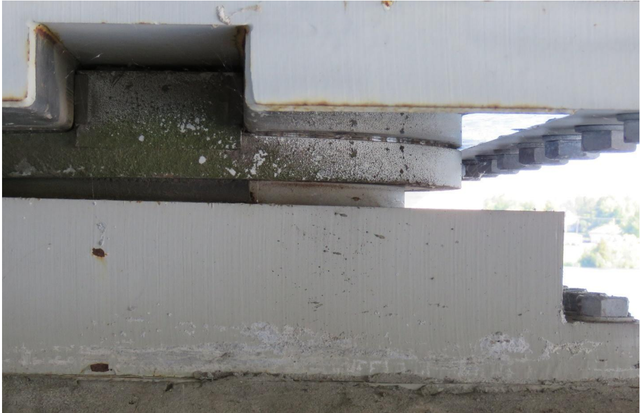
Figure A.12 (e) Disc Bearing
