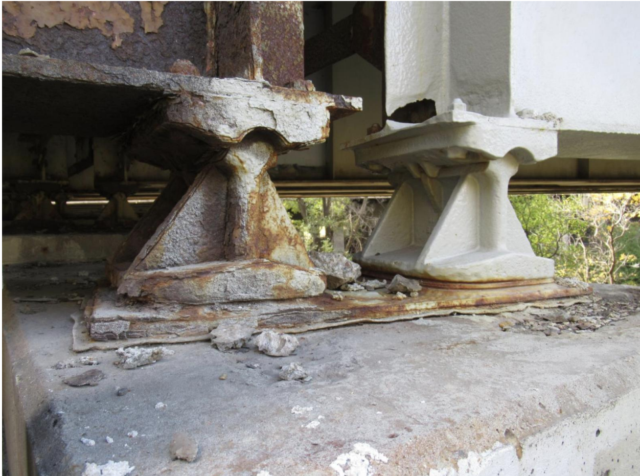
Figure A.12 (f) Rocker Bearings
