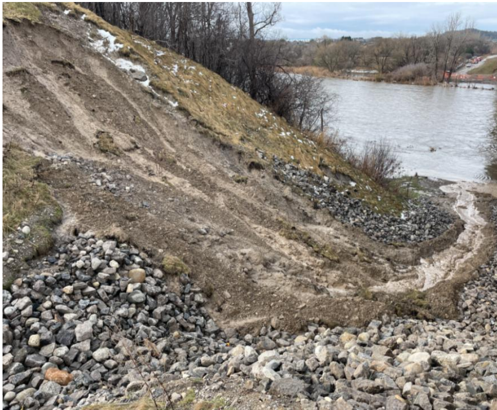
Figure A.9 (e) Slope Protection
