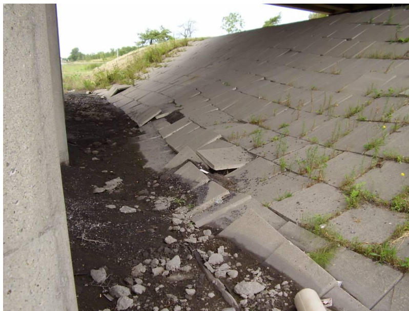
Figure A.9 (g) Precast Concrete Slope Protection
