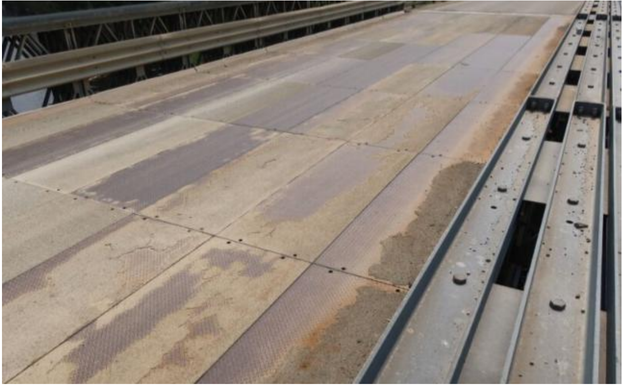
Figure A.8 (t) Steel Deck – Friction Coat Break Down
