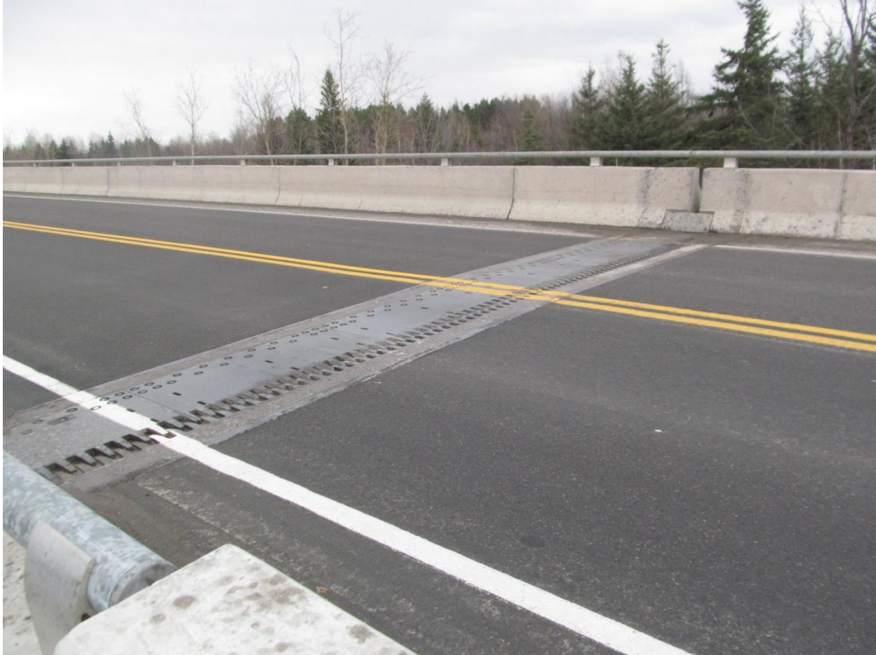
Figure A.11 (a) Finger Plate Expansion Joint
