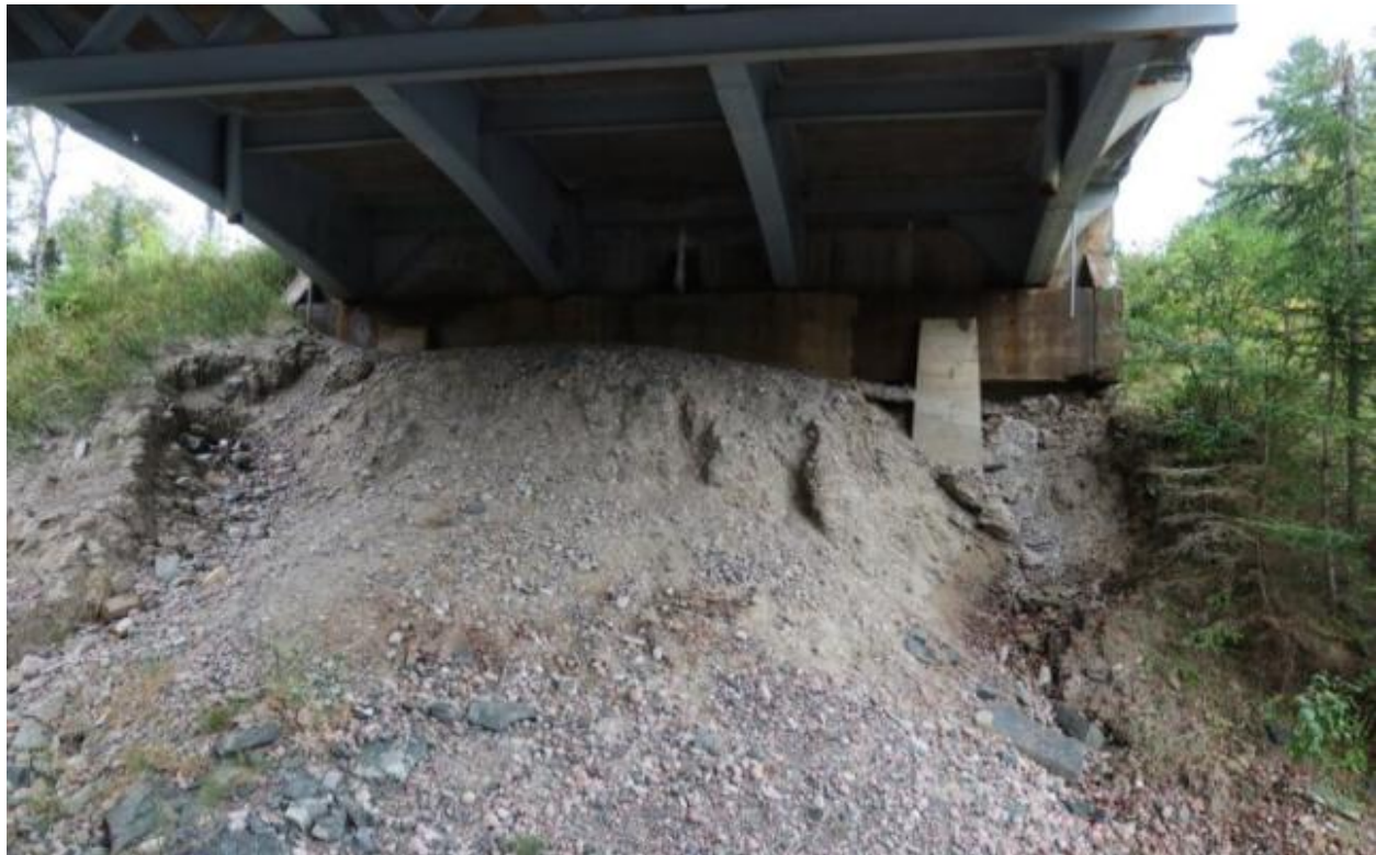
Figure A.9 (c) Embankments
