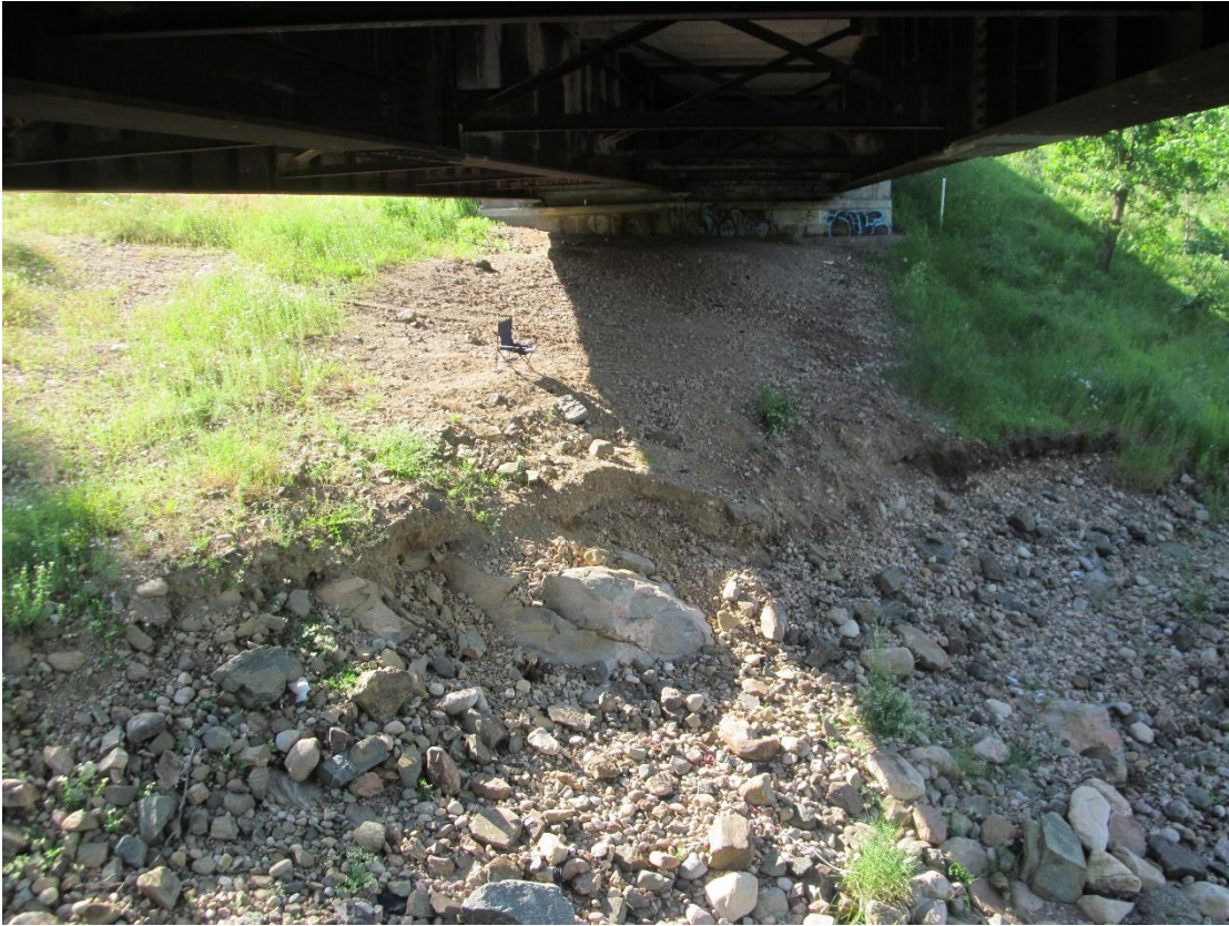
Figure A.9 (b) Embankment
