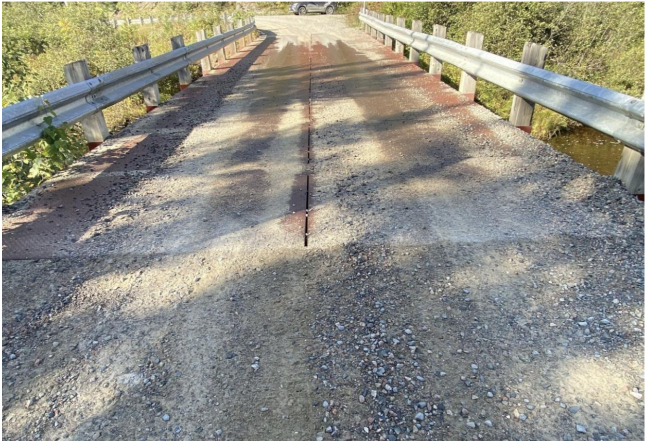
Figure A.8 (s): Steel Deck
