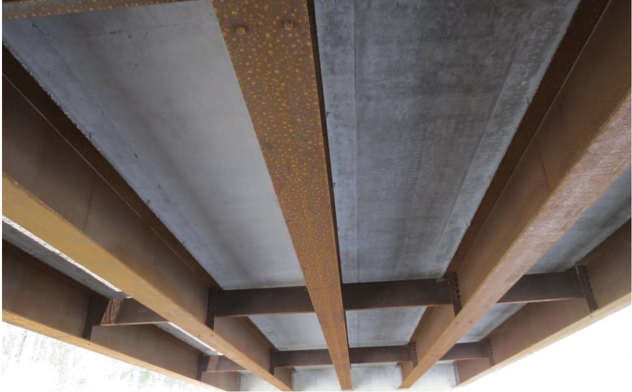
Figure A.8 (i) Soffit of a Thin Slab
