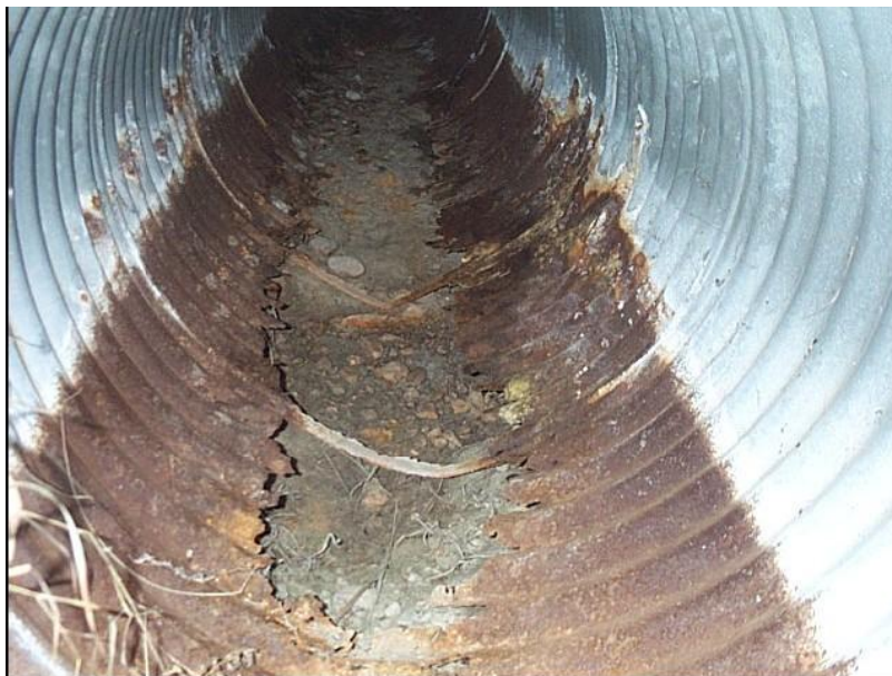
Figure A.7 (e) Multi-Plate Pipe Arch
