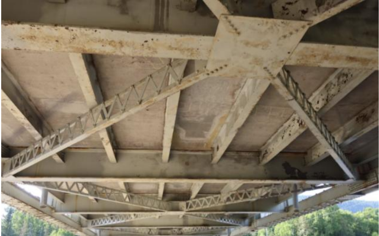
Figure A.5 (a) Steel Beam Bracing
