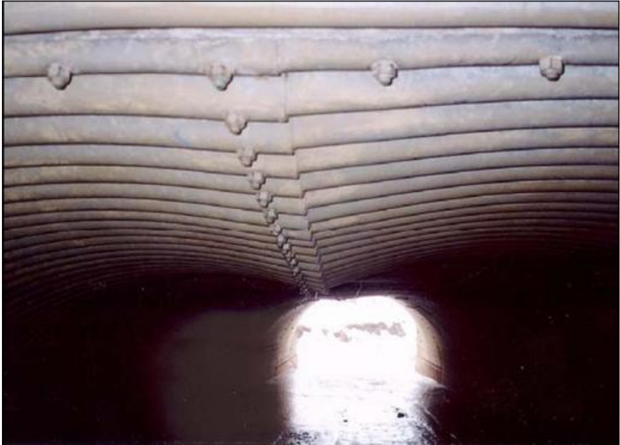
Figure A.7 (b) Multi-Plate Pipe Arch
