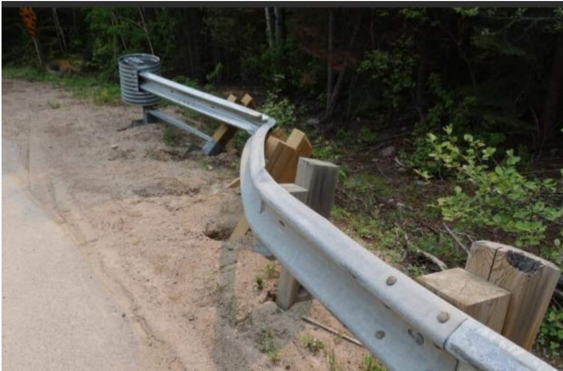
Figure A.3 (h) Steel Flex Beams
