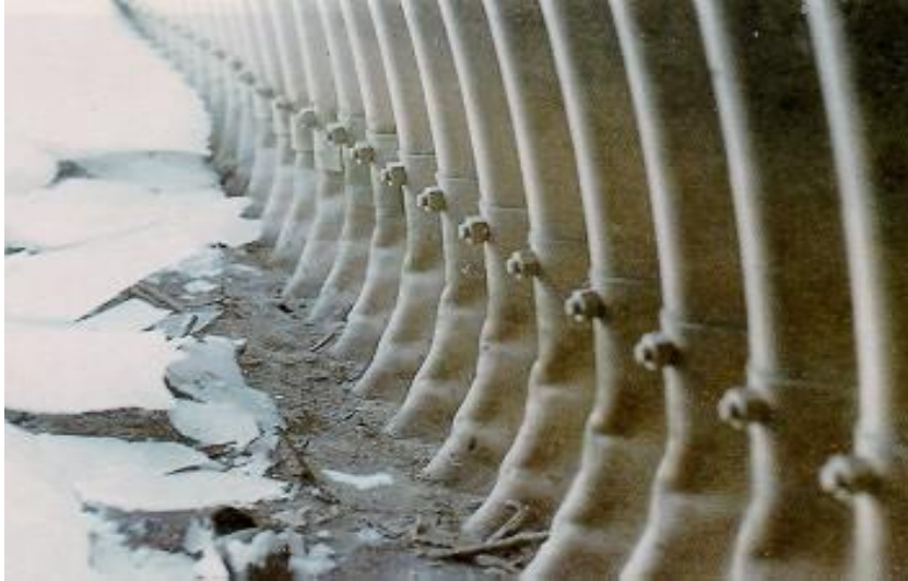
Figure A.7 (a) Multi-Plate Pipe Arch
