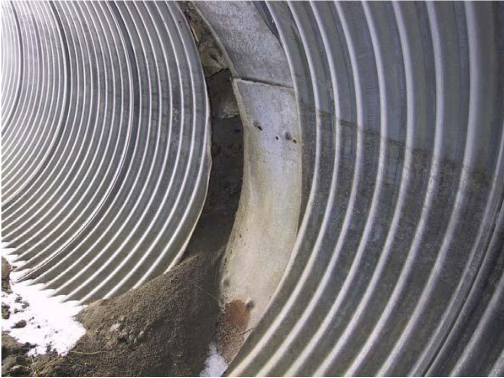
Figure A.7 (bc) Multi-Plate Pipe Arch
