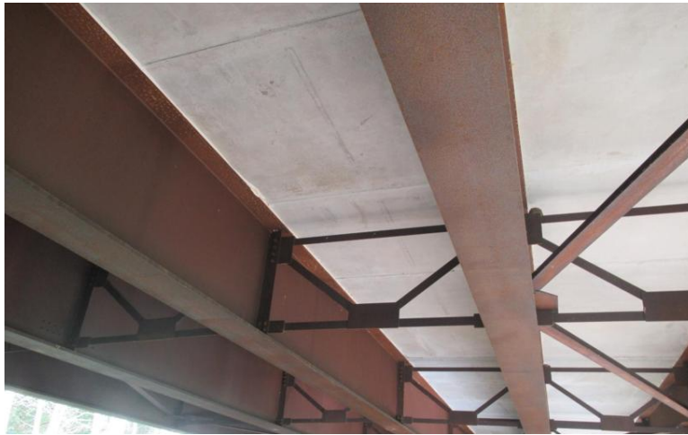
Figure A.5 (b) Intermediate Diaphragms
