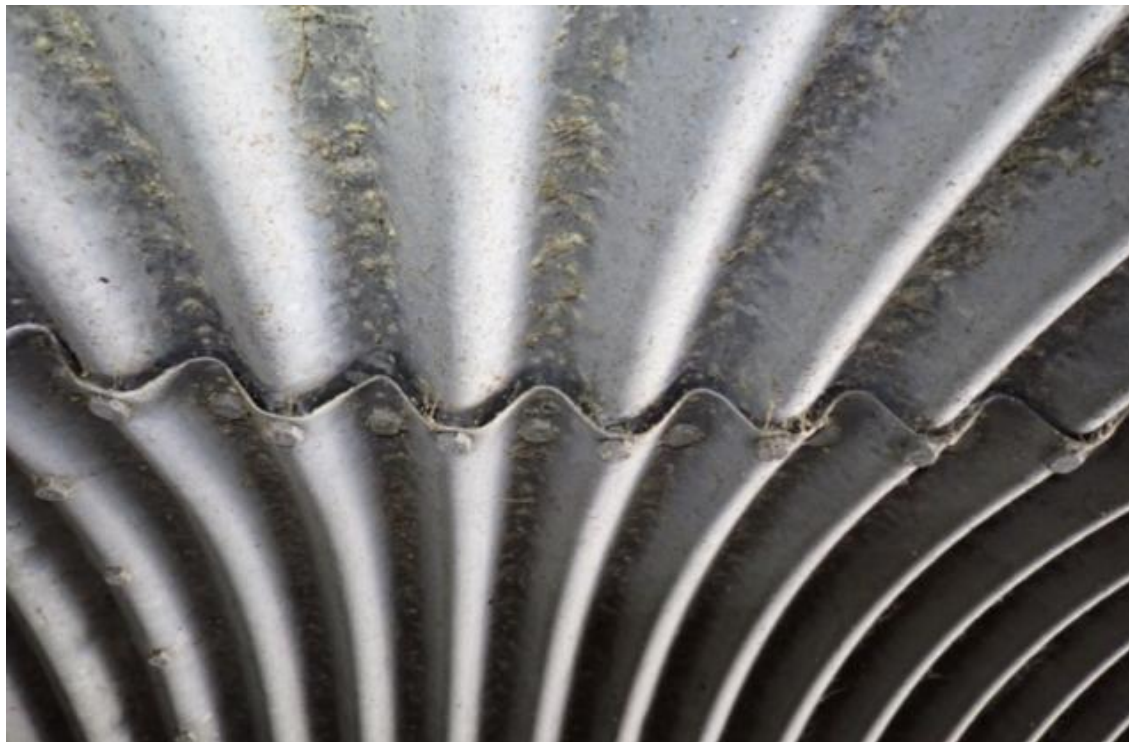
Figure A.7 (f) Multi-plate Pipe Arch
