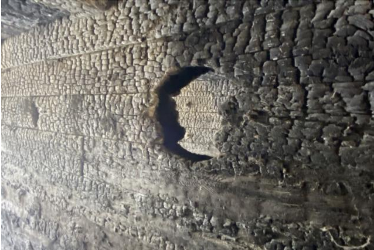
Figure A.7 (h) Wood Culvert Barrel
