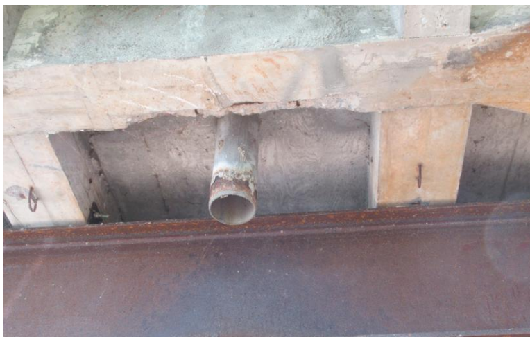
Figure A.8 (e) Steel Deck Drain
