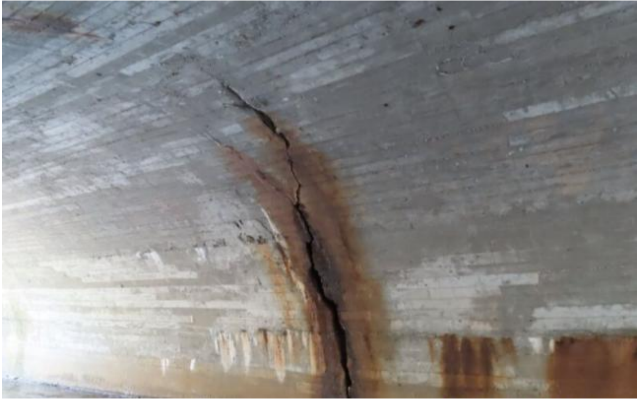
Figure A.7 (g) Concrete Arch Culvert
