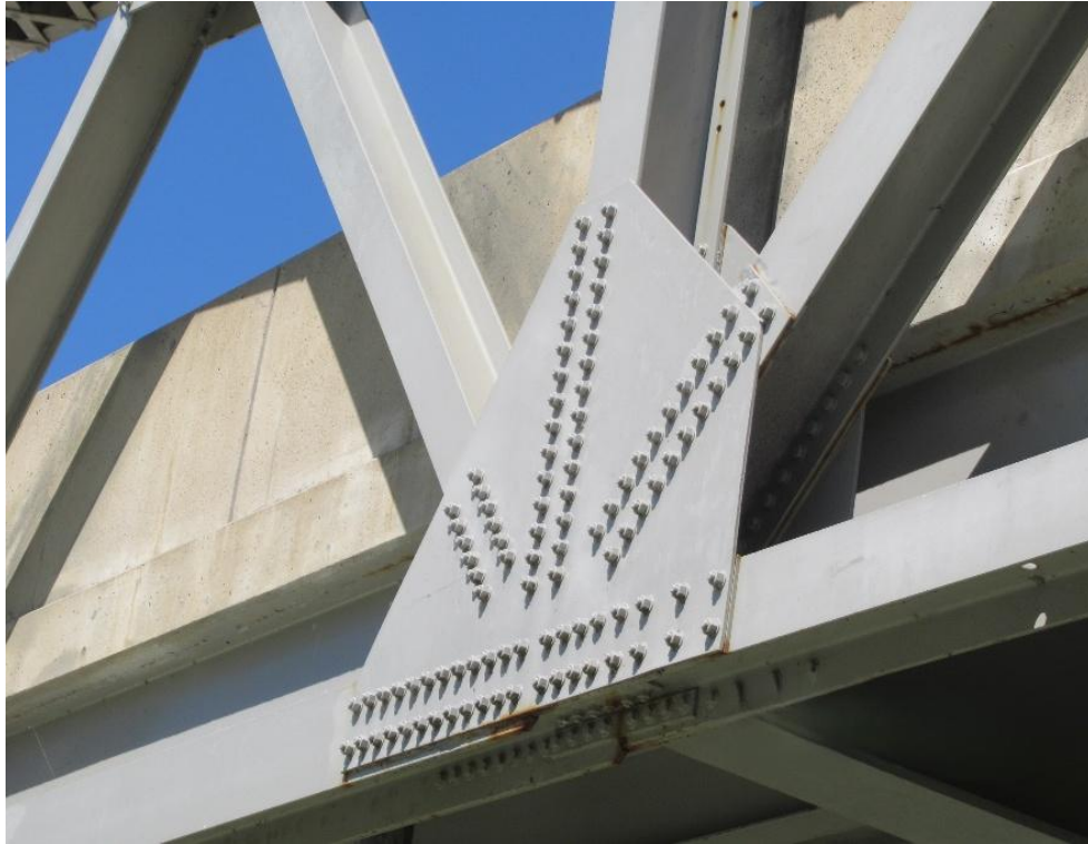
Figure A.6 (c) Coating of Connection - Bottom Chord
