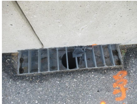
Figure A.8 (g) Deck Drain with Basin
