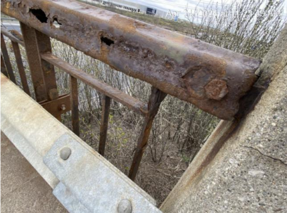
Figure A.3 (f) Steel Railing
