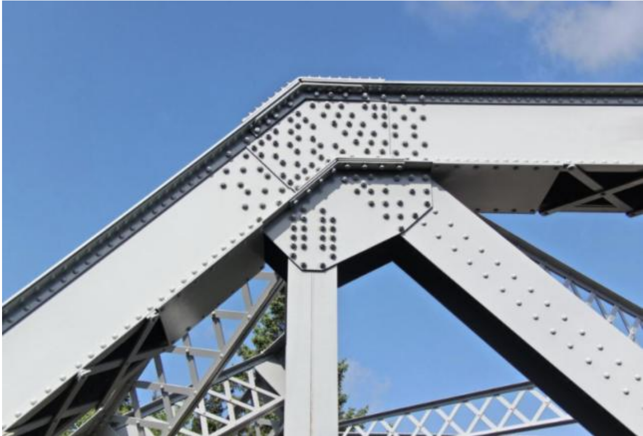
Figure A.6 (a) Coating of Through Truss
