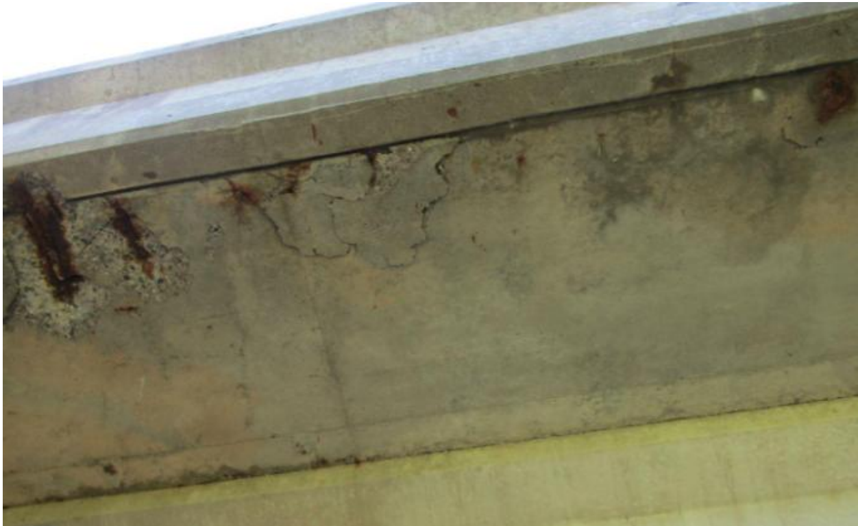
Figure A.8 (o) Deck Soffit Exterior – Thin Slab
