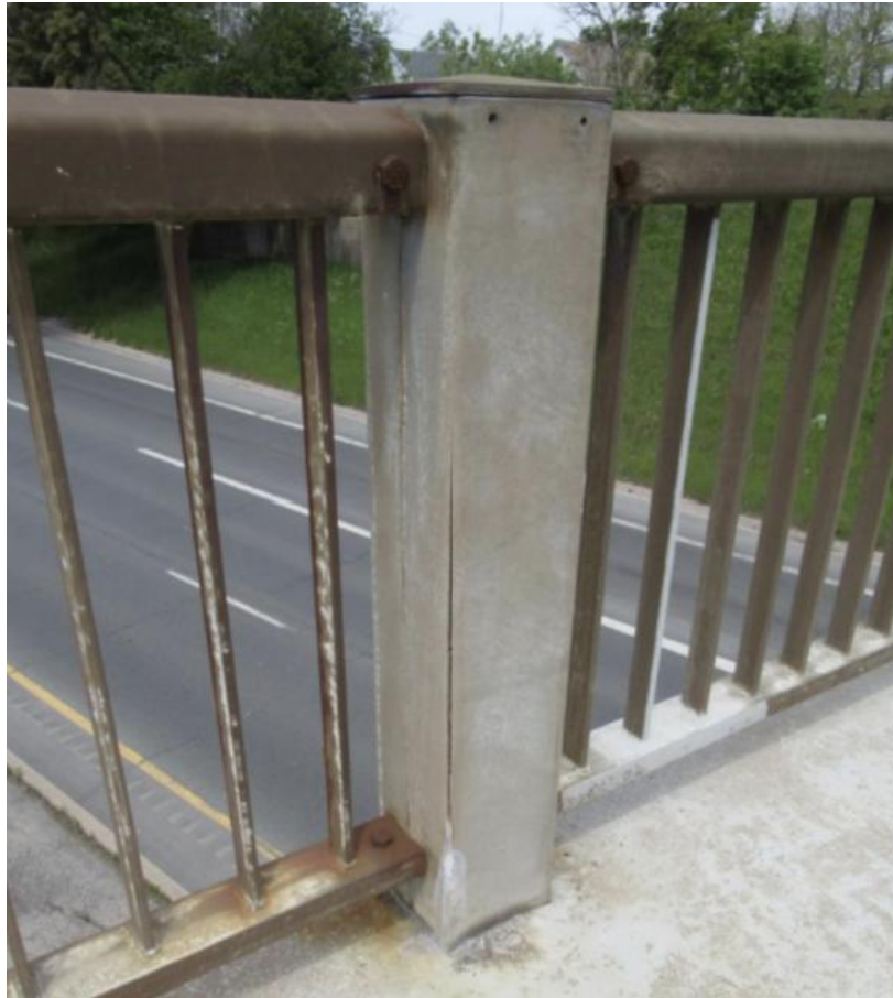
Figure A.3 (e) Steel Railing with Steel Posts (Concrete-Filled)
