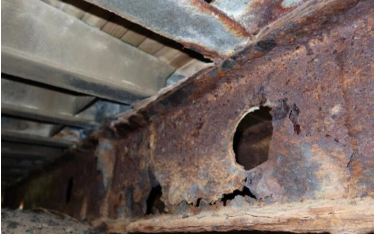
Figure A.4 (a) Beam Girder/MLE - Stringer
