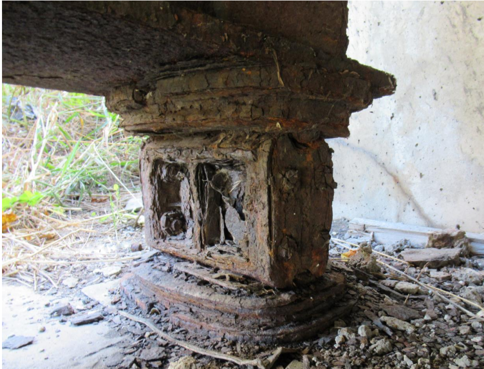
FigureA.1 (m) Steel Rocker Bearing
