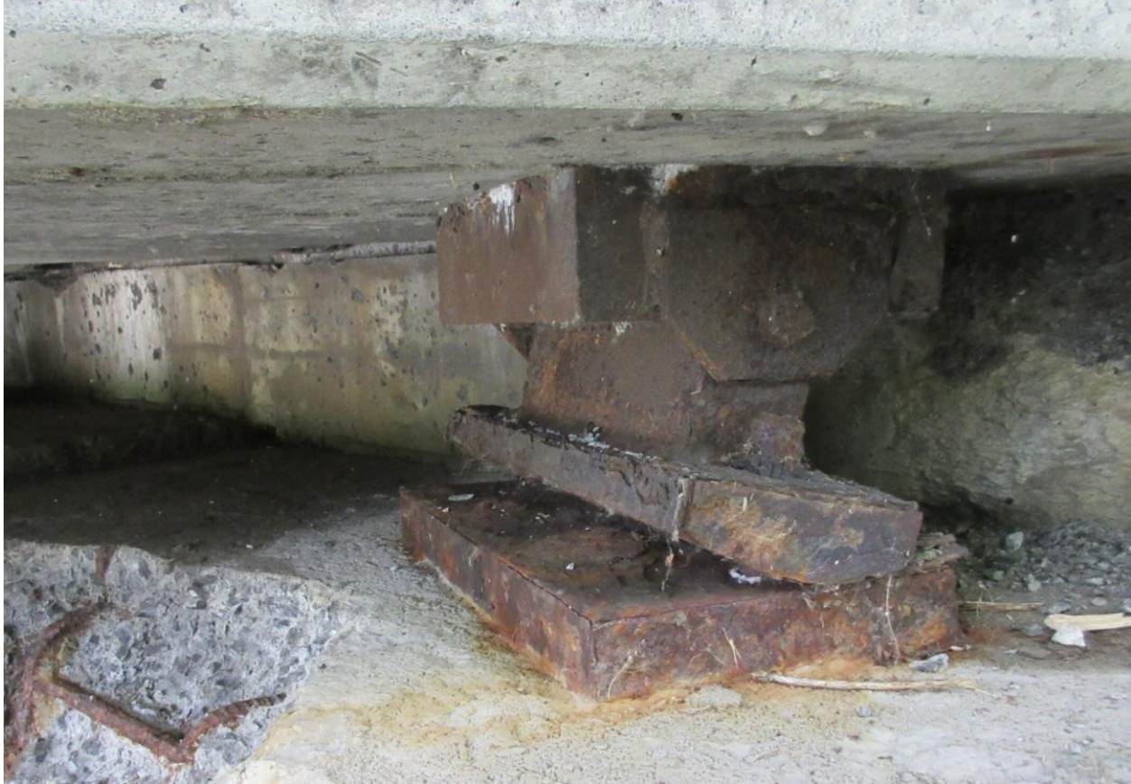
FigureA.1 (I) Steel Rocker Bearing
