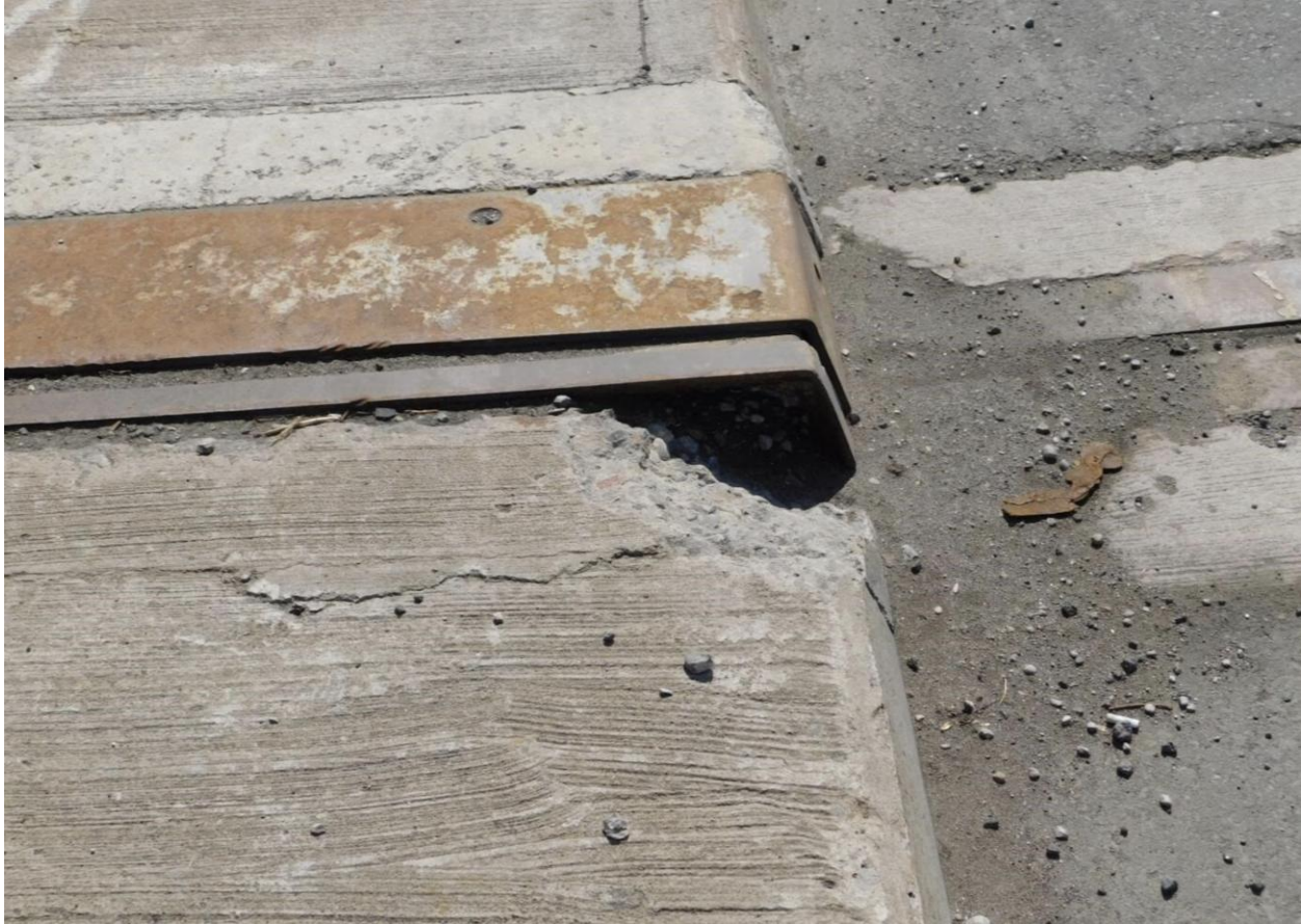
FigureA.2 (b) Approach: Concrete Sidewalk
