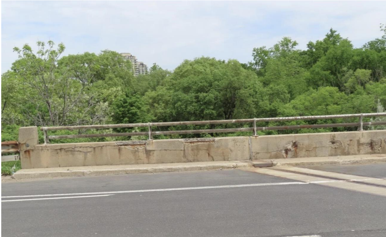
Figure A.3 (a) Parapet Wall
