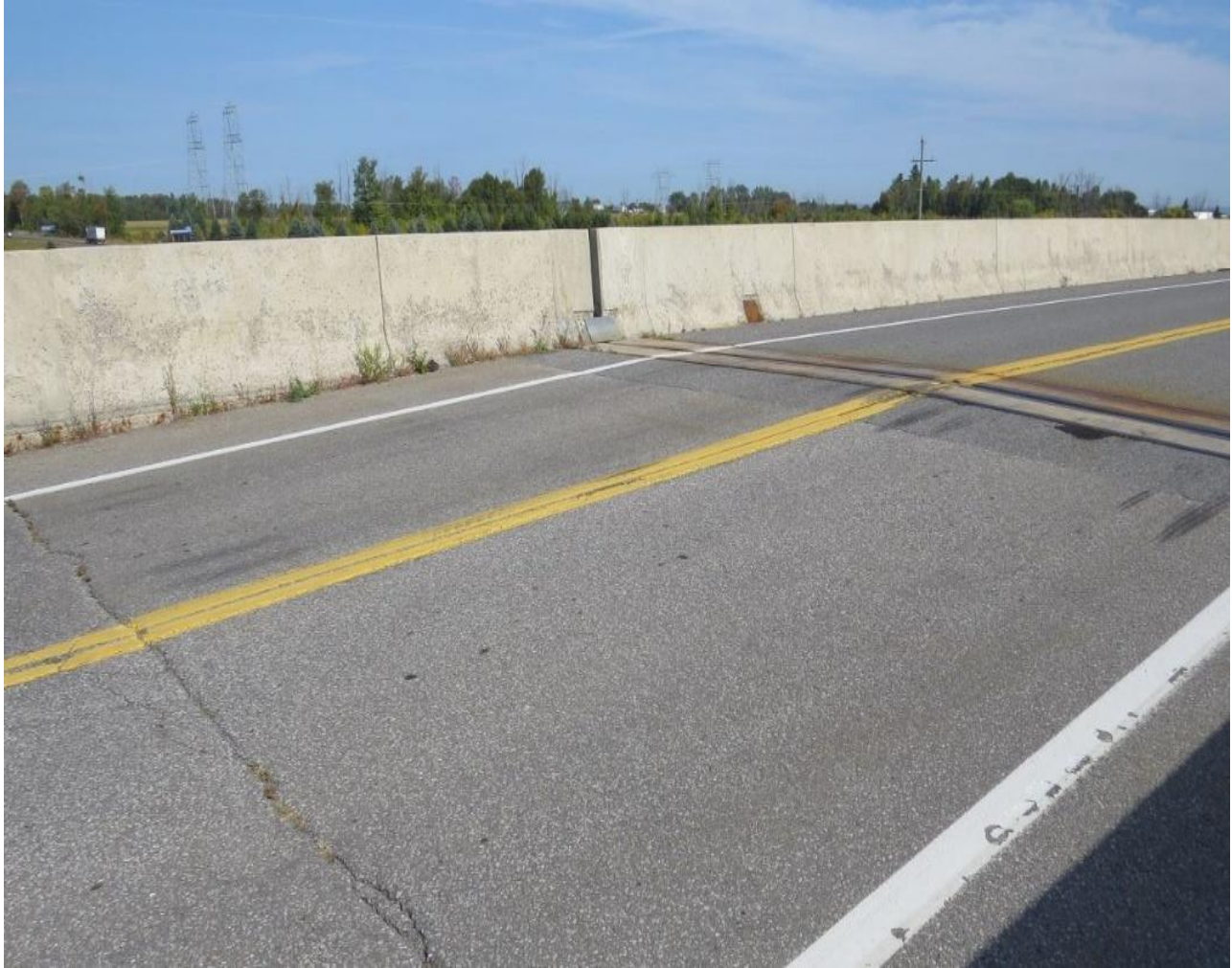
Figure A.2 (a) Concrete Approach Slab
