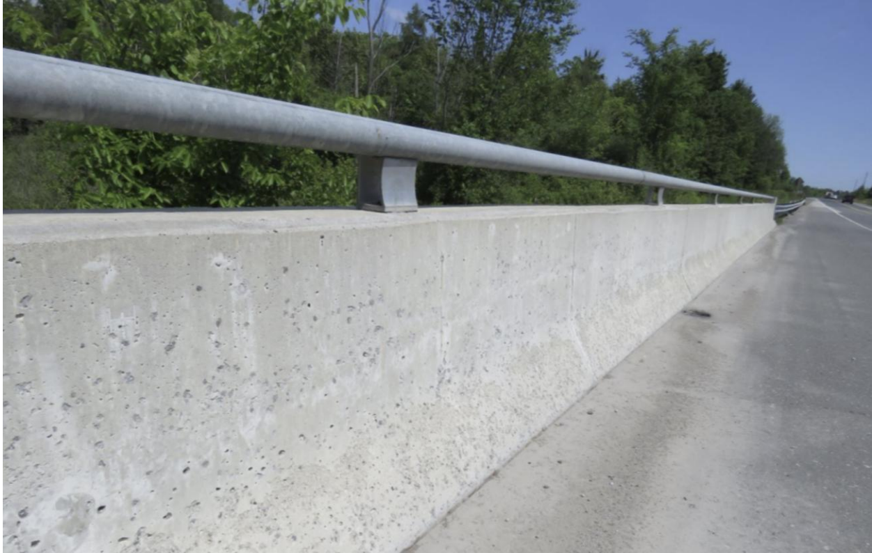
FigureA.3. (b) Barrier Wall
