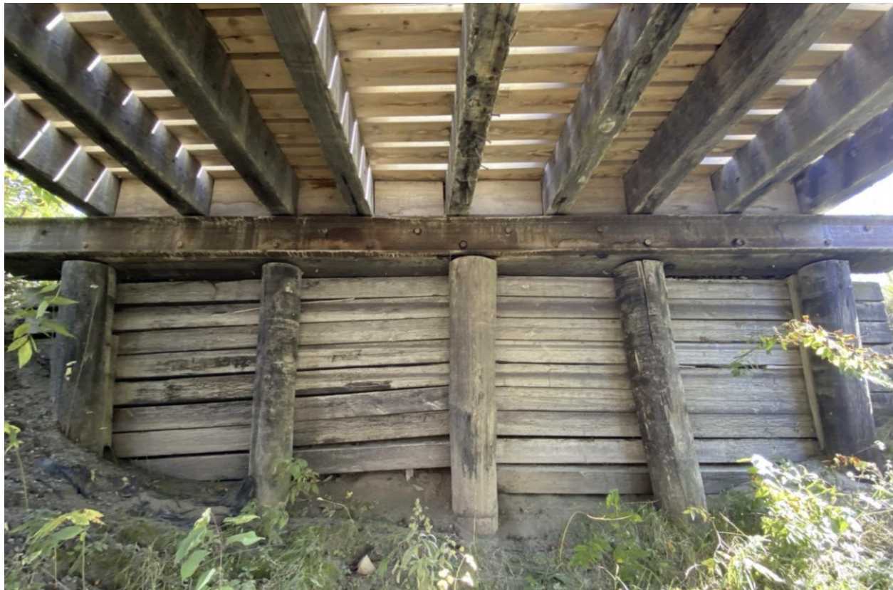
Figure A.1 (b) Wood Lagging – Abutment Wall
