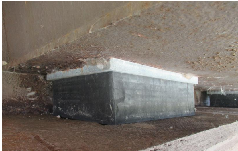
Figure A.1 (j) Laminated Elastomeric Bearing
