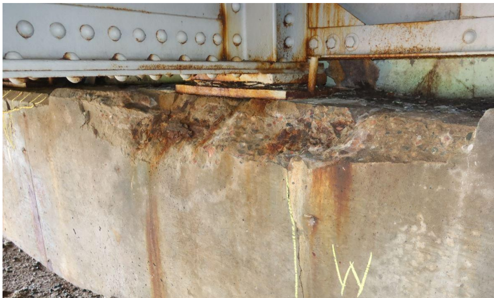
Figure A.1 (e) Concrete Abutment Wall
