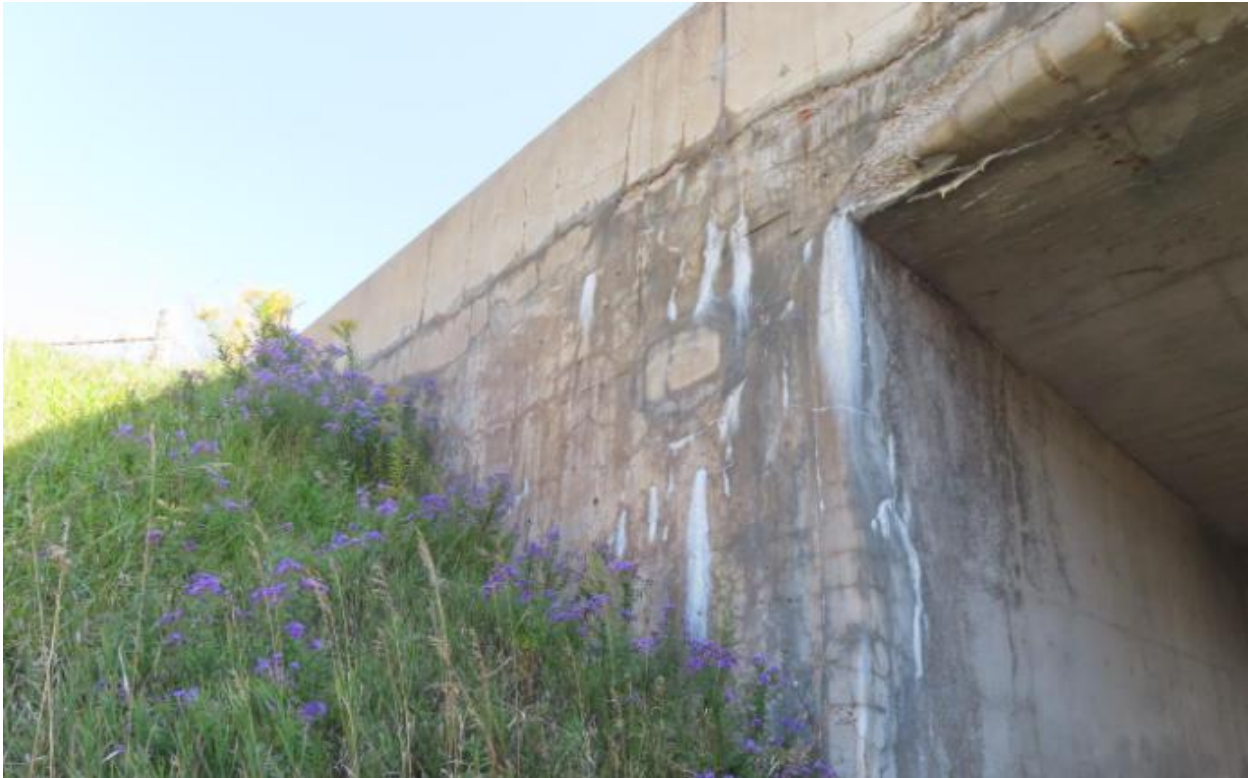
Figure A.1 (a) Concrete Wingwall.
