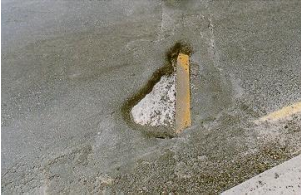
Figure 2.5.8.7 Severe Pothole
