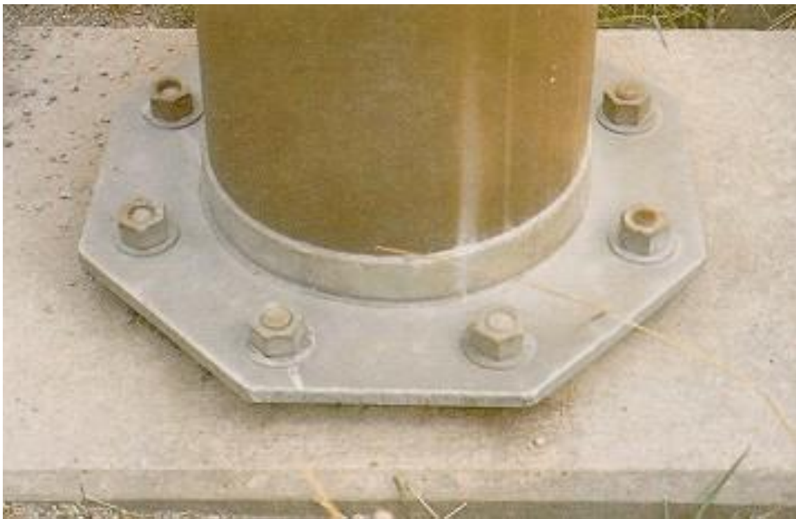
Figure 2.5.7.1 Light Corrosion
