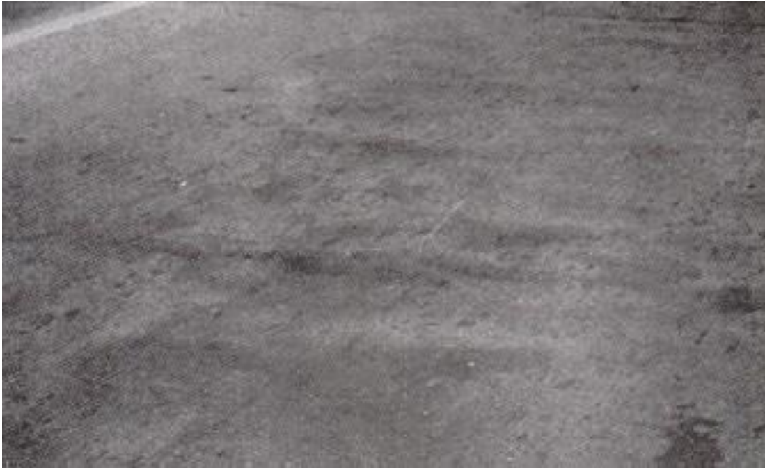
Figure 2.5.8.6 Severe Rippling
