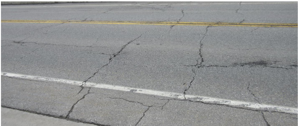
Figure 2.5.8.4 Map Cracking
