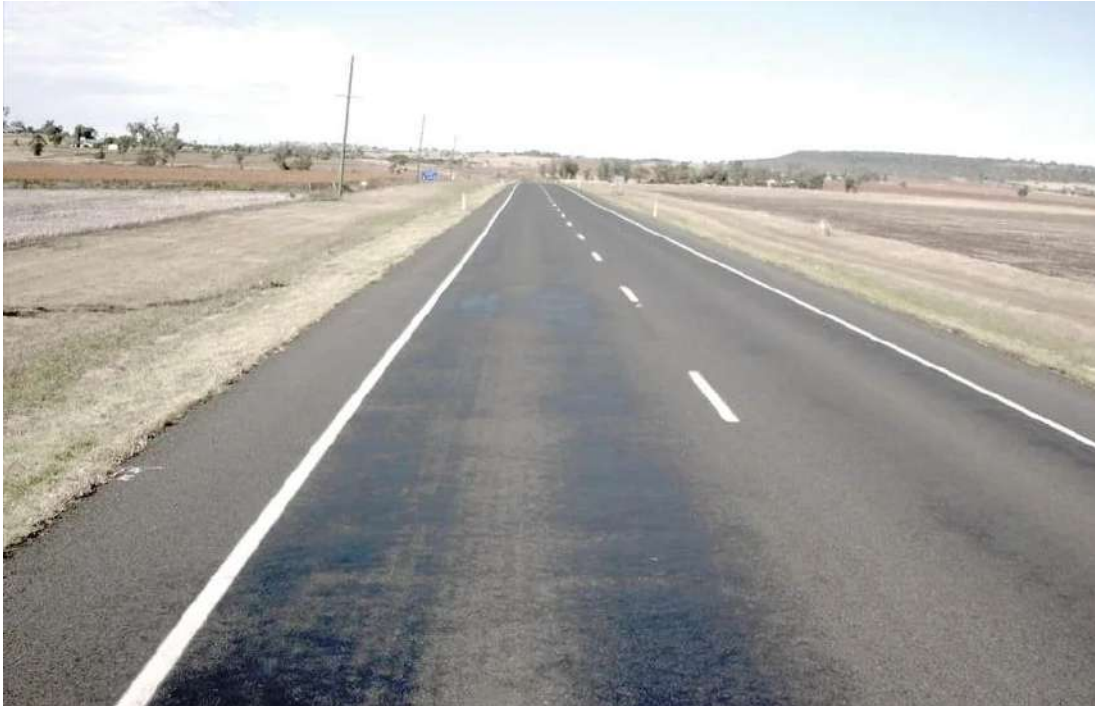
Figure 2.5.8.9 Severe Flushing
