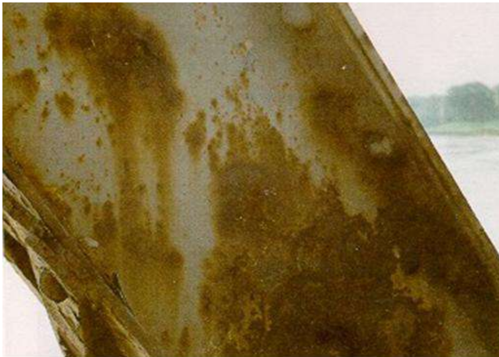
Figure 2.5.5.5 Undercutting
