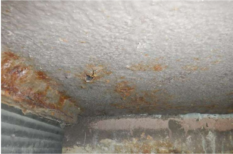
Figure 2.5.5.4 Chemical Attack
