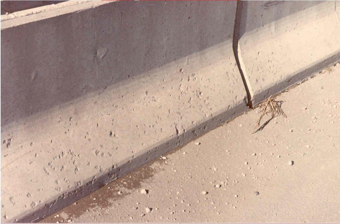
FIGURE 1. Example of Light Scaling
