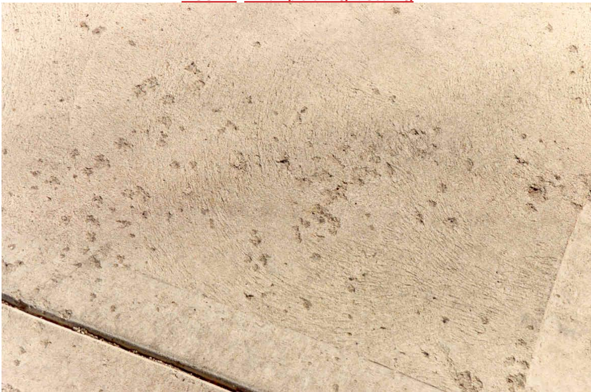
FIGURE 2. Example of Light Scaling
