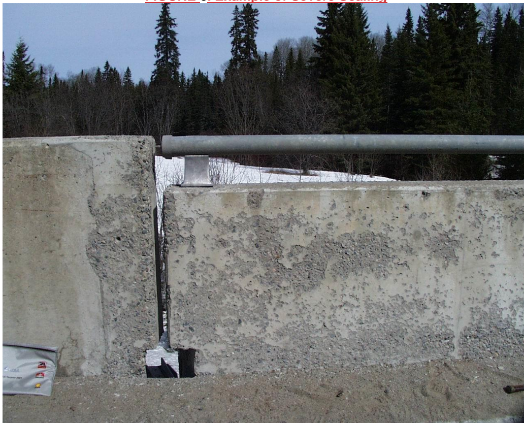
FIGURE 6. Example of Severe Scaling
