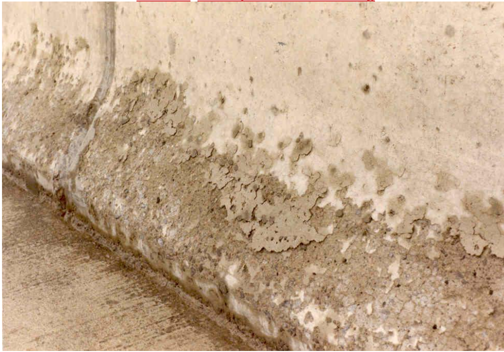
FIGURE 6. Example of Severe Scaling
