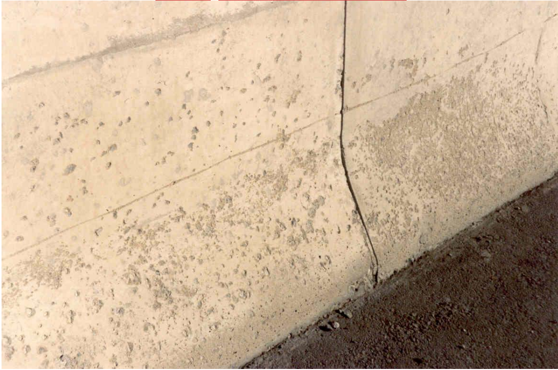
FIGURE 3. Example of Medium Scaling
