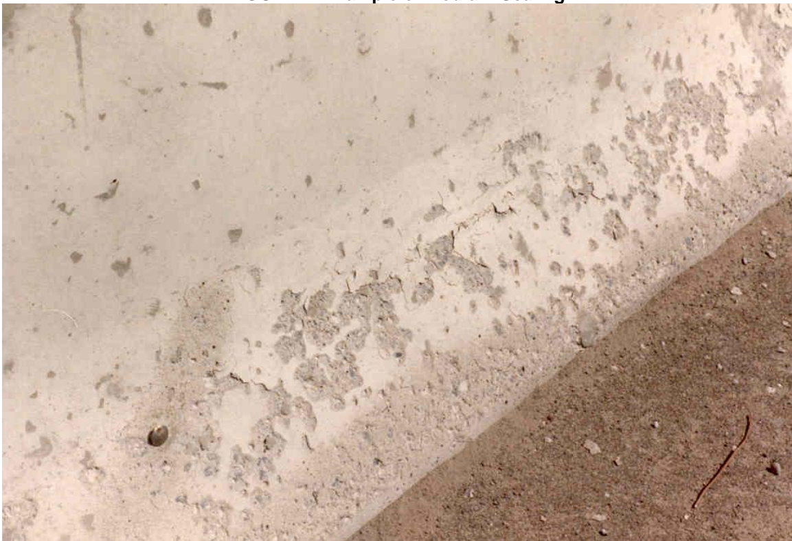
FIGURE 4. Example of Medium Scaling
