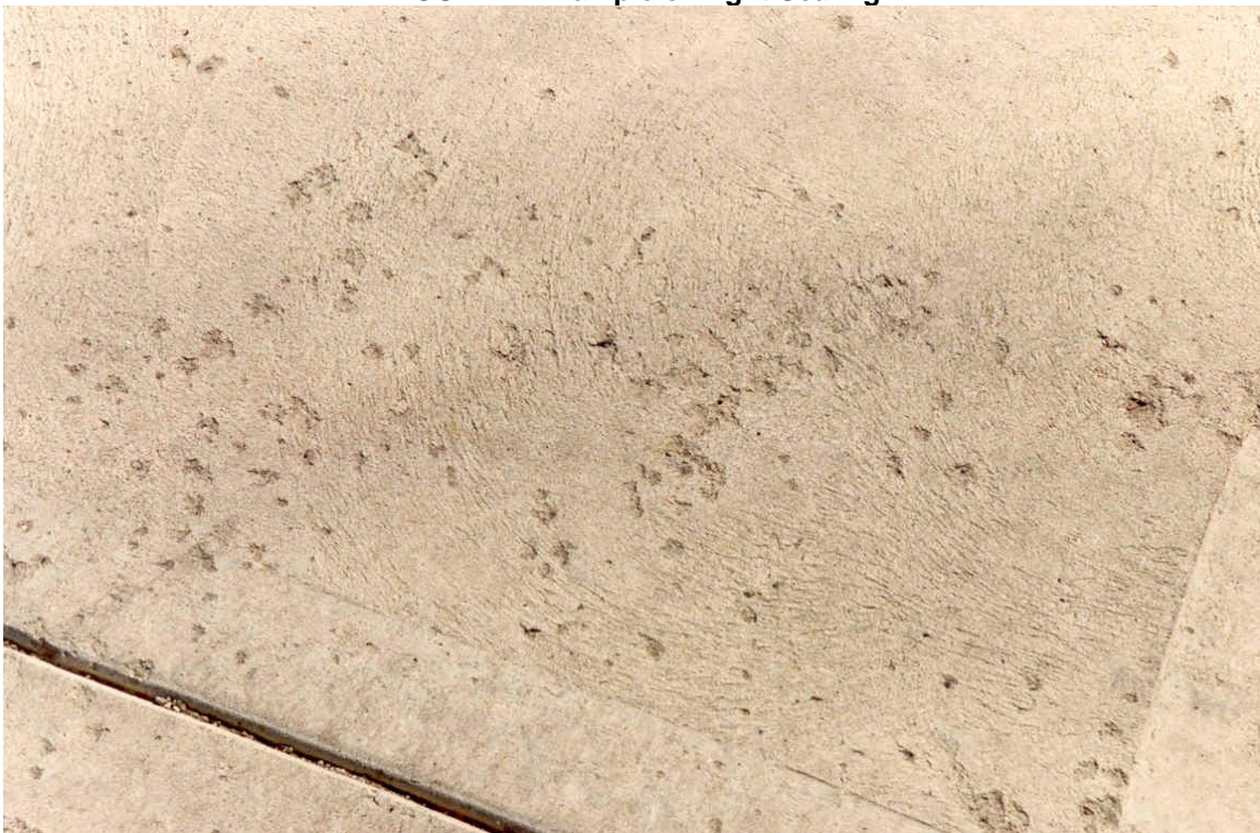
FIGURE 2. Example of Light Scaling
