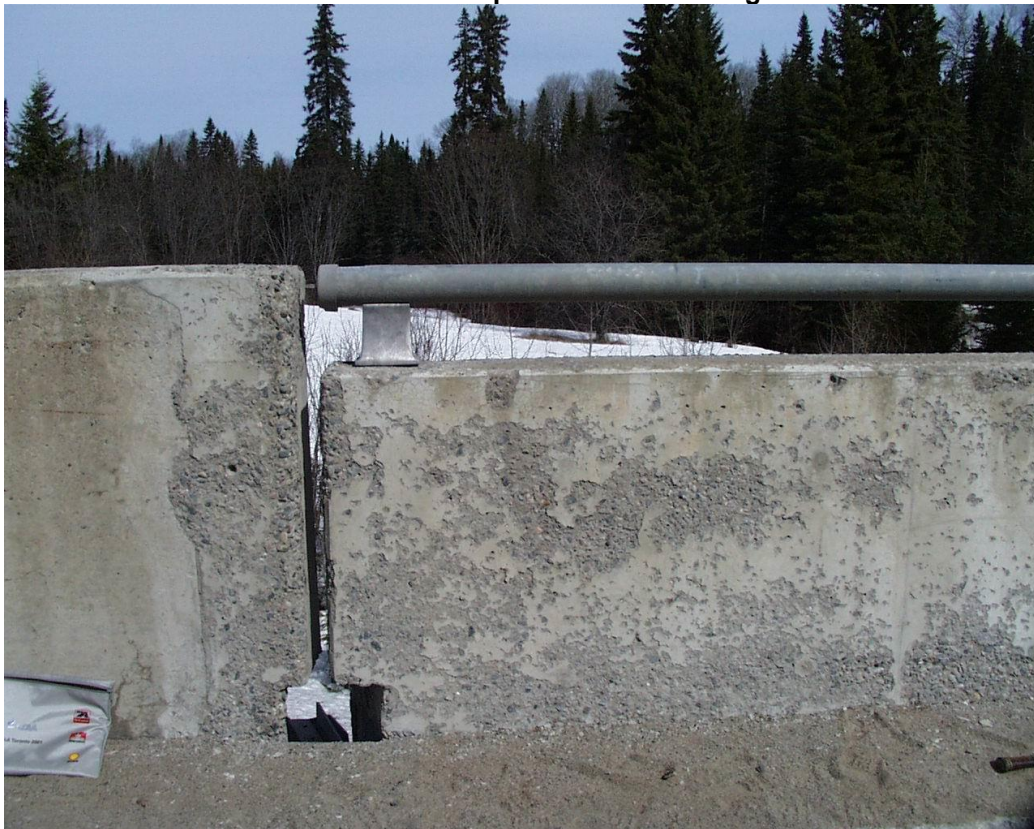
FIGURE 6. Example of Severe Scaling
