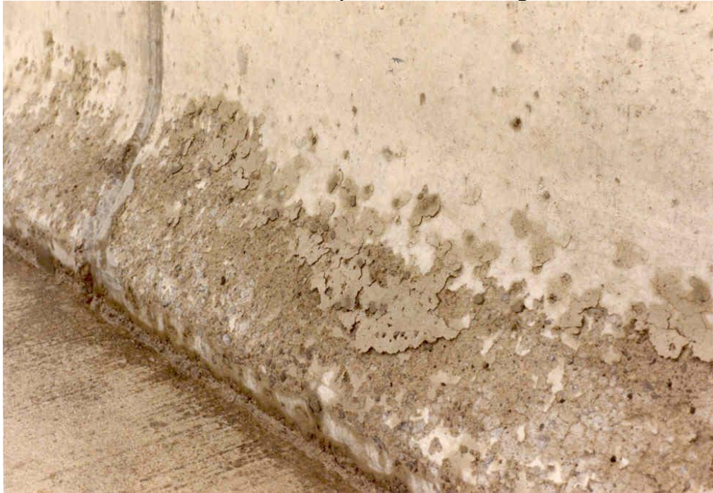
FIGURE 6. Example of Severe Scaling
