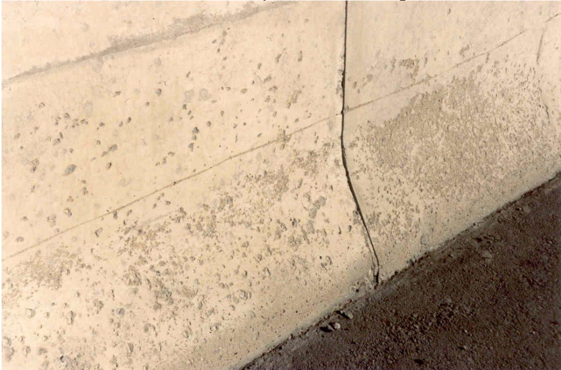
FIGURE 3. Example of Medium Scaling
