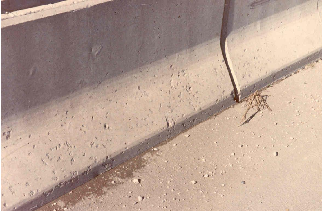
FIGURE 1. Example of Light Scaling
