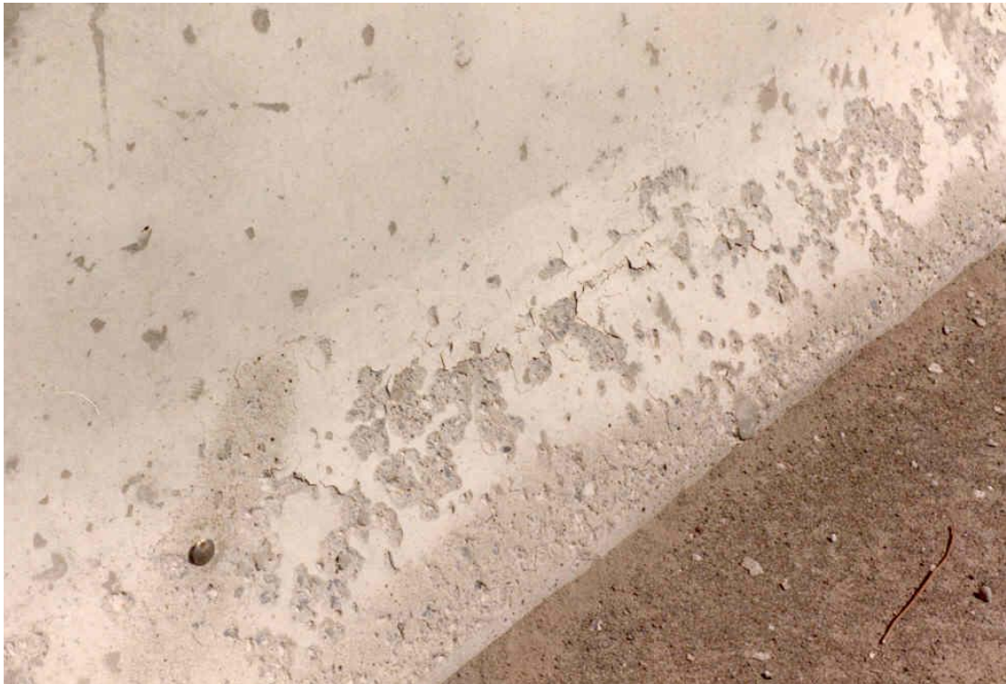
FIGURE 4 Example of Medium Scaling
