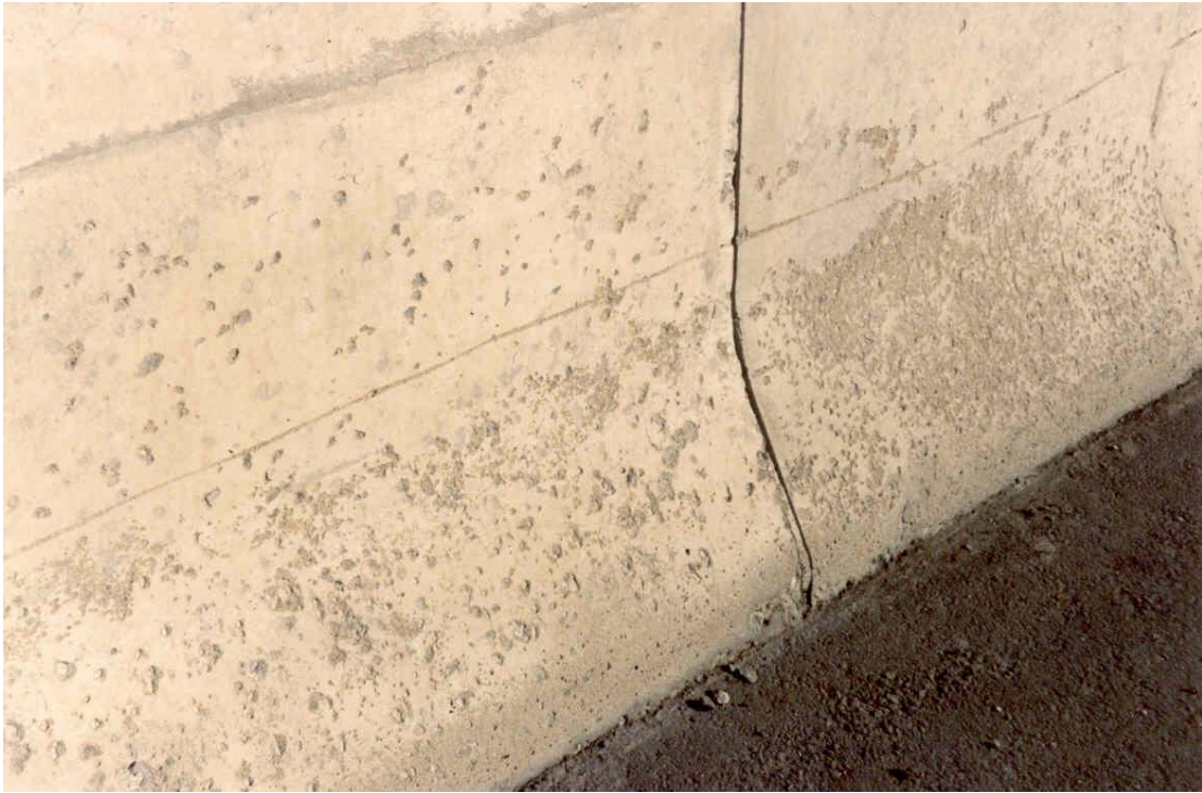
FIGURE 4 Example of Medium Scaling
