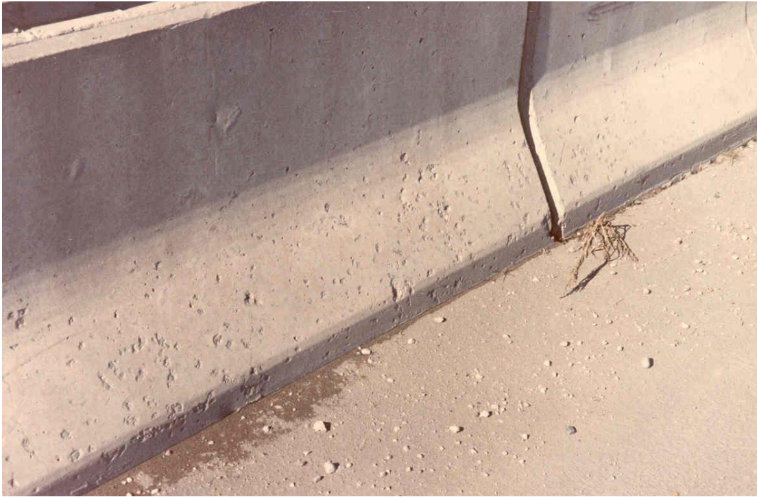
FIGURE 2 Example of Light Scaling
