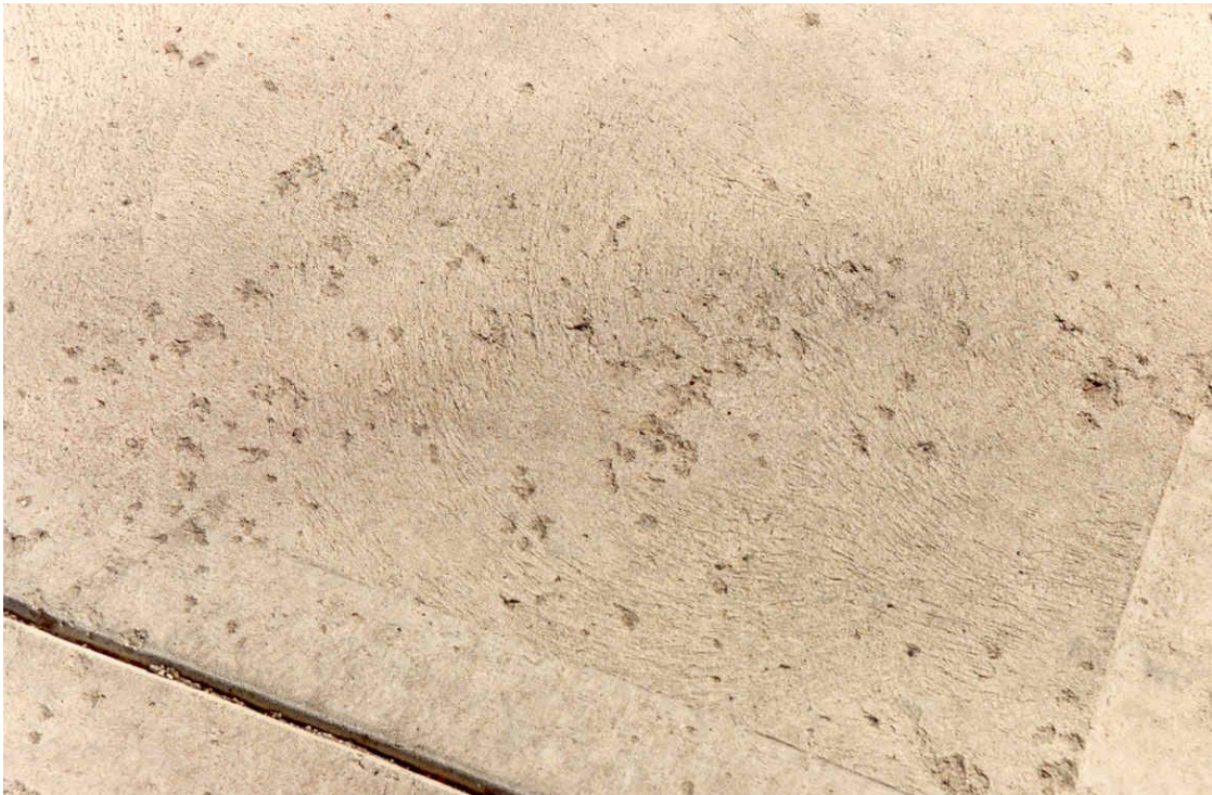
FIGURE 2 Example of Light Scaling
