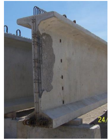
Figure 57 – Web Spall
