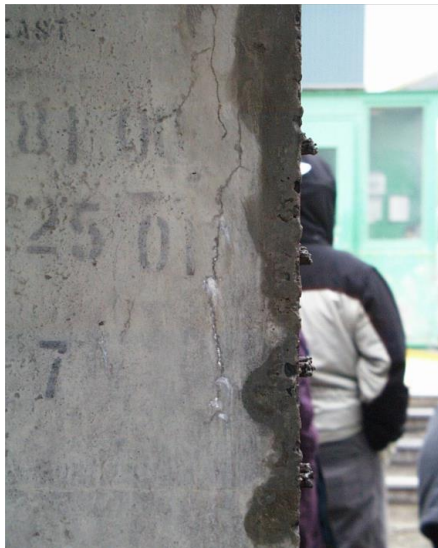
Figure 58 – Web Cracking
