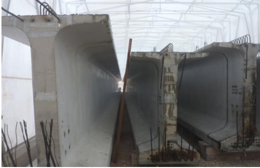
Figure 43 – Moist Curing
