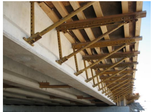
Figure 49 – Deck Formwork
