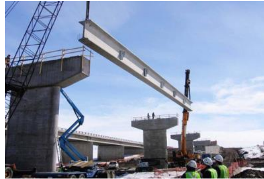
Figure 46 – Girder Erection
