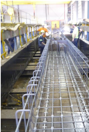
Figure 33 – Box Rebar Cage
