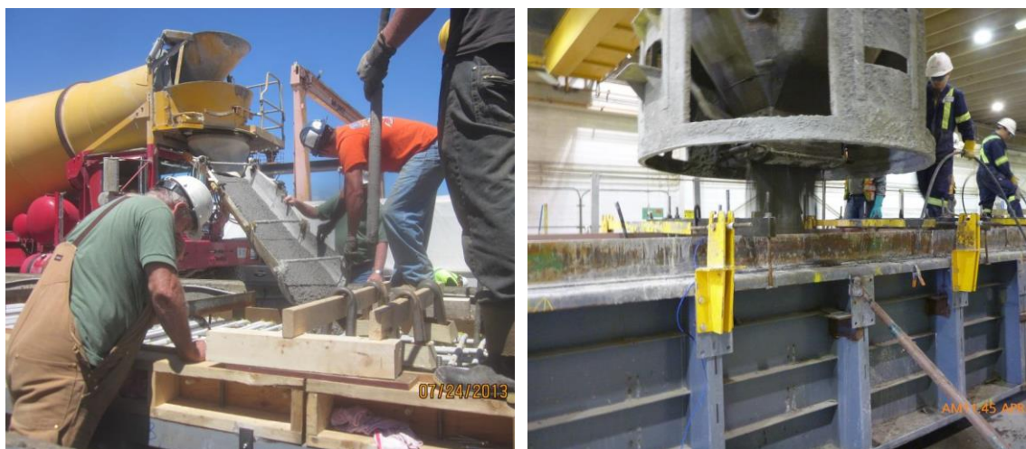
Figure 50 – Casting Concrete, Outdoor and Indoor
