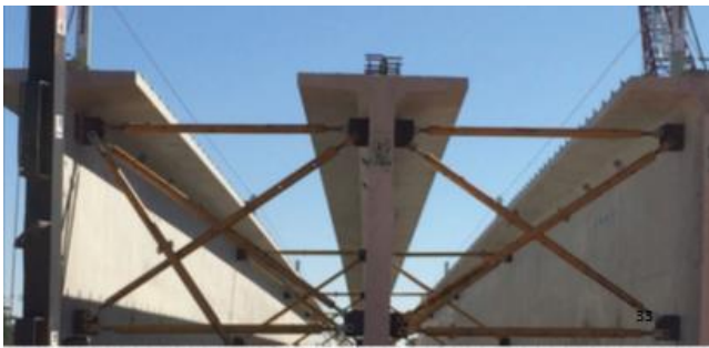
Figure 48 – Girder Temporary Bracing
