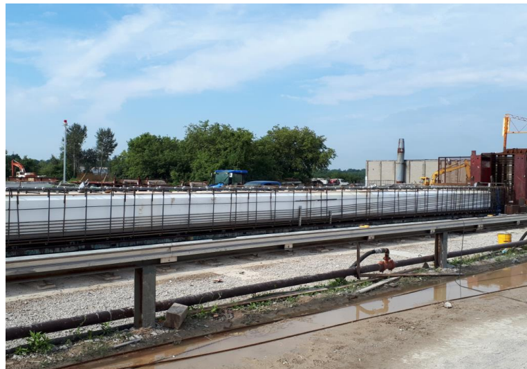
Figure 34 – Box Girder Void
