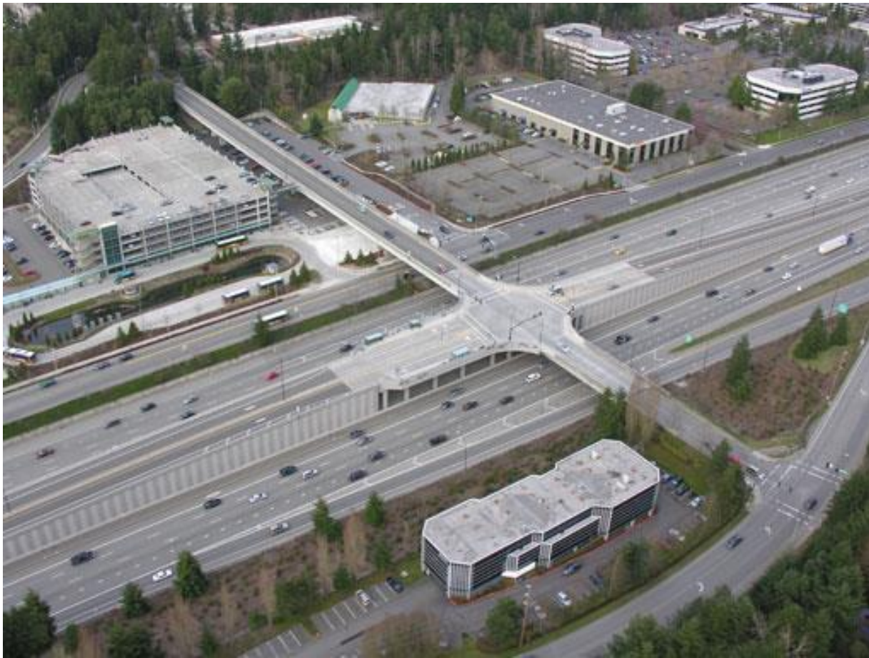
Figure 12.4.2 Aerial View of HOV Direct Access Ramps
