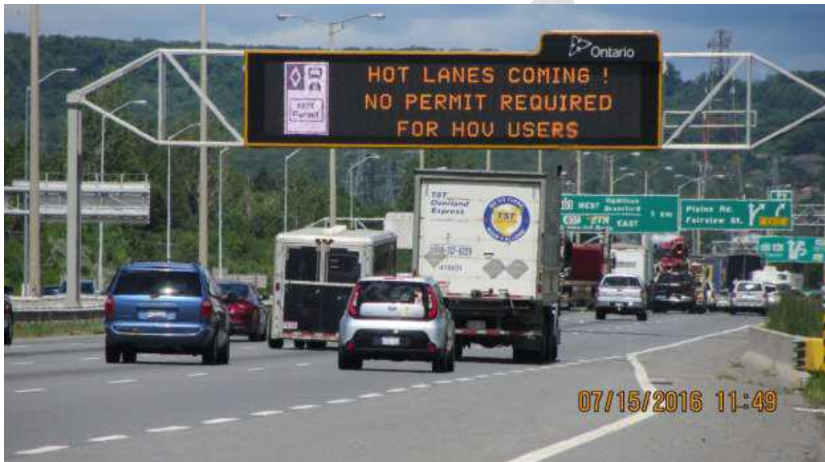
Figure 12.1.2 HOT Lanes Pilot Digital Message Signs
