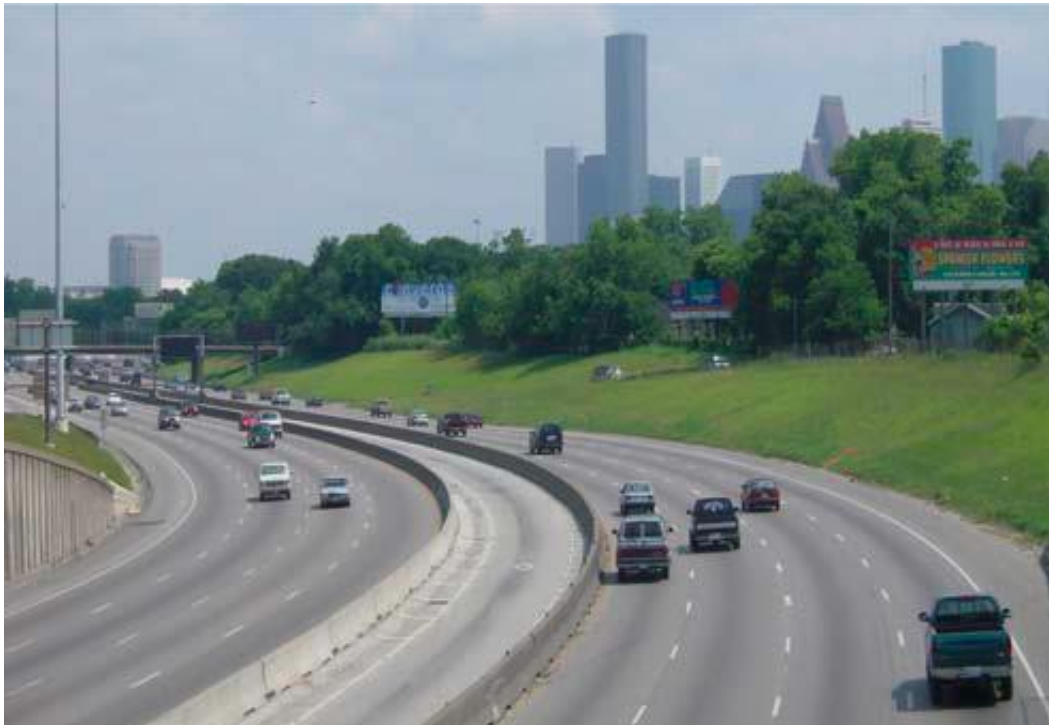
Figure 12.11.3 Freeway Median Busway (Interstate 45, Huston, Texas)
