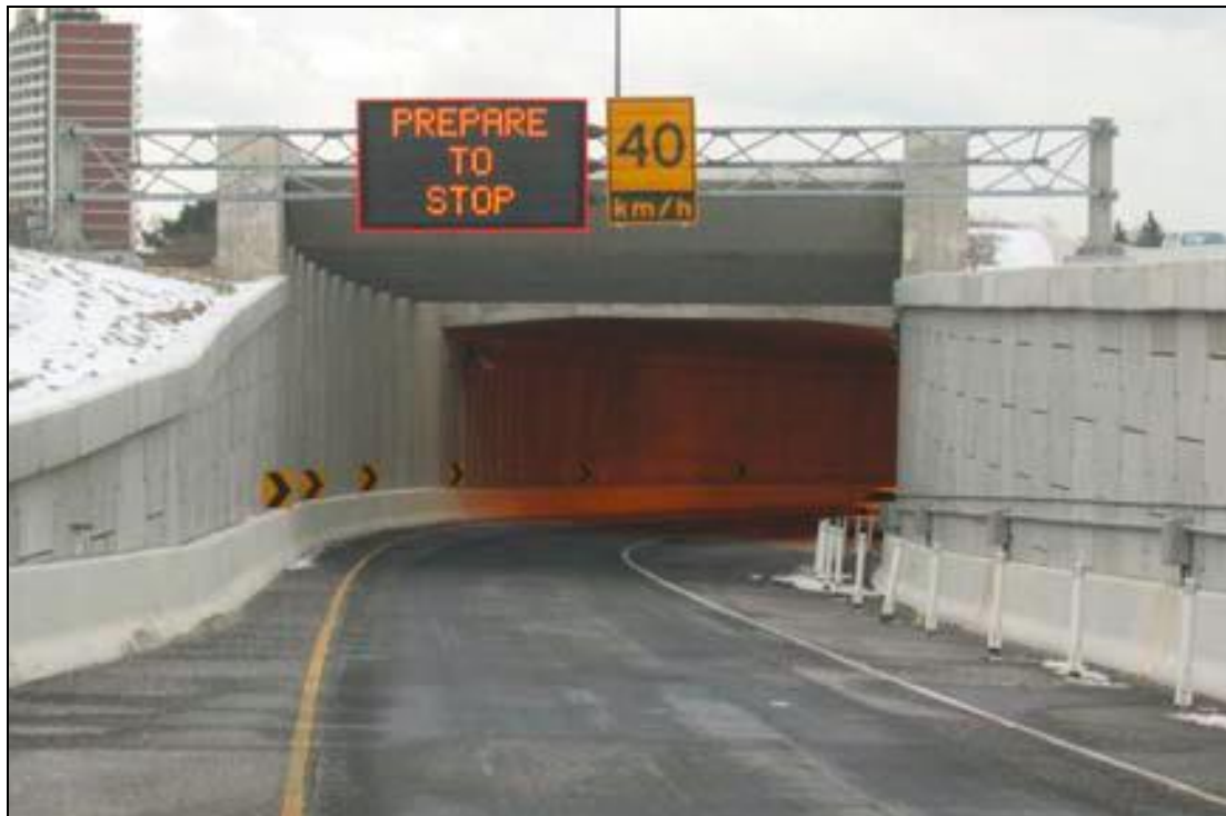
Figure 12.7.1 Highway 404 Tunnel Automated Warning Message
