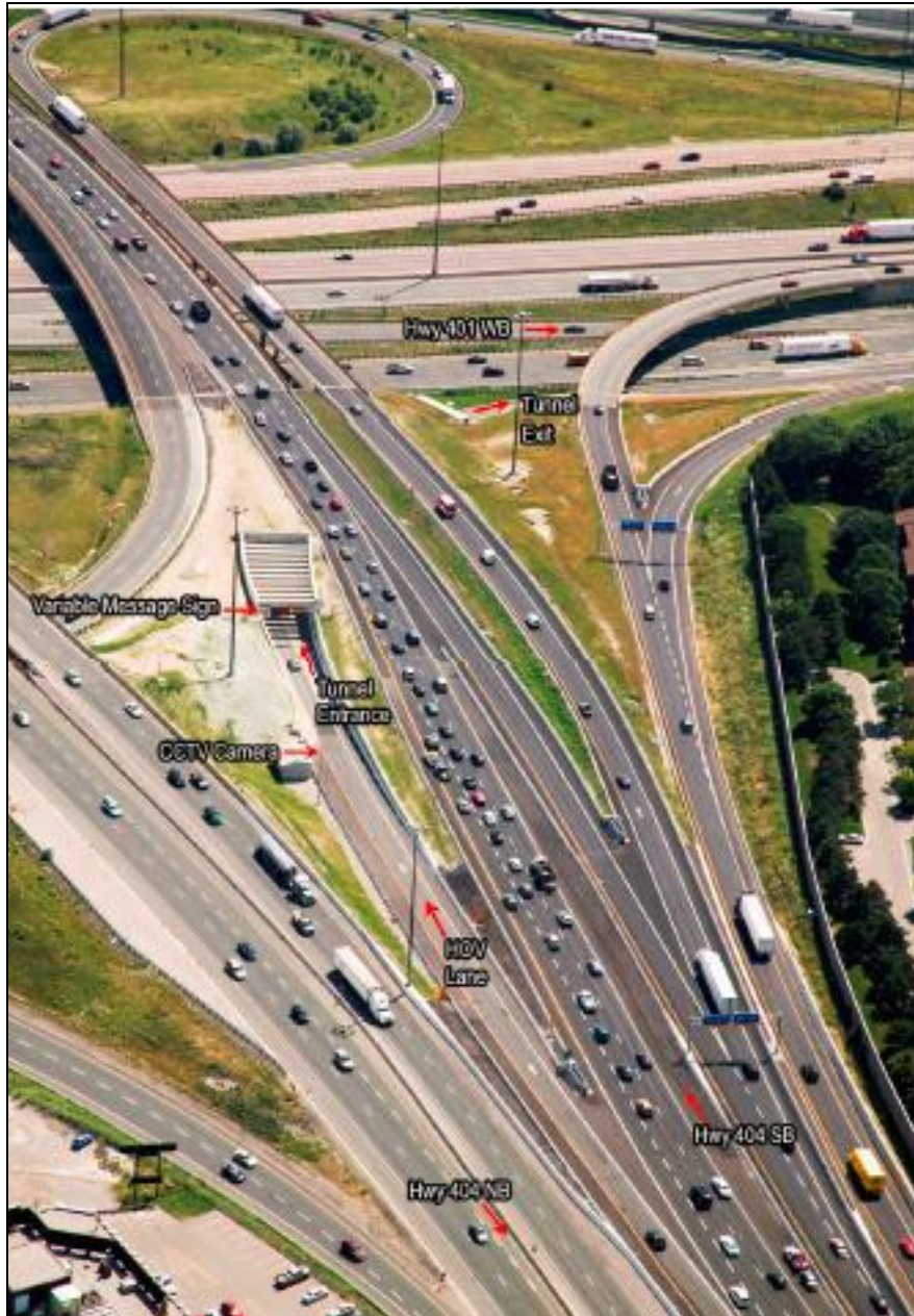
Figure 12.7.3 Highway 404 and Highway 401 VMS at Tunnel Entrance
