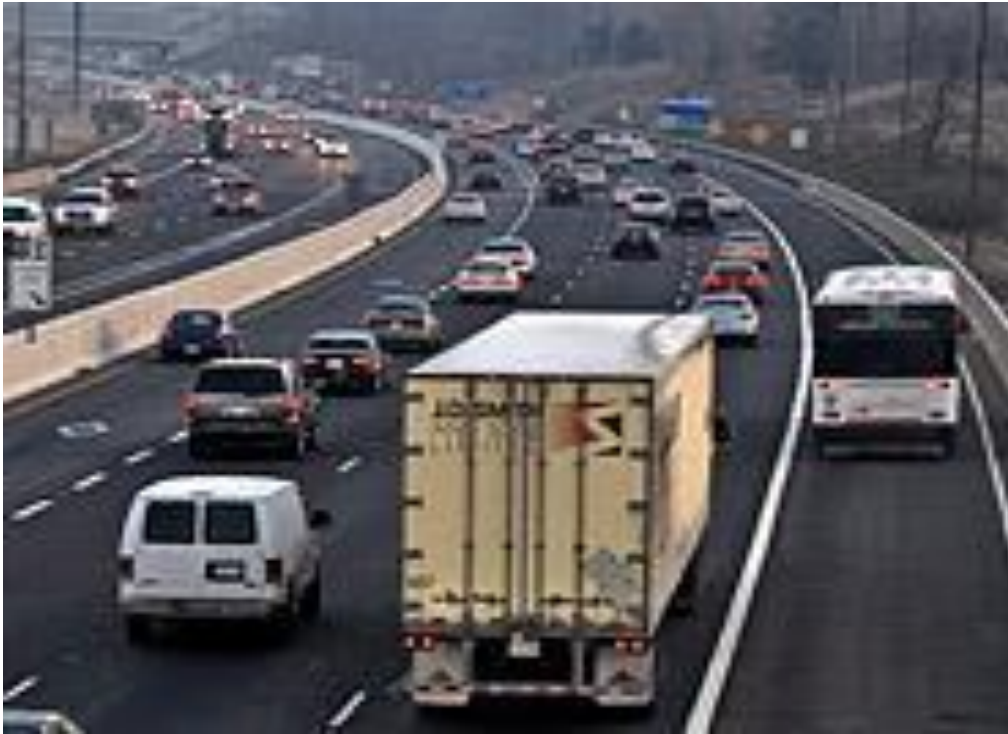
Figure 12.11.14 Bus ByPass Shoulders
