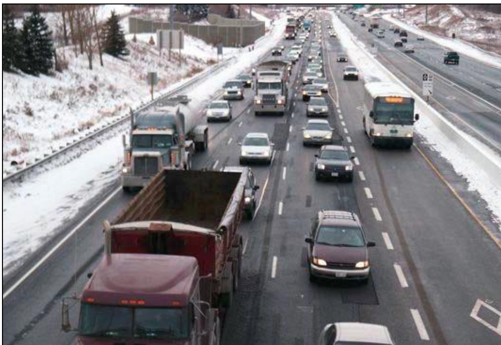
Figure 12.11.15 Mississauga Transit including Bus ByPass Shoulders on Highway 403
