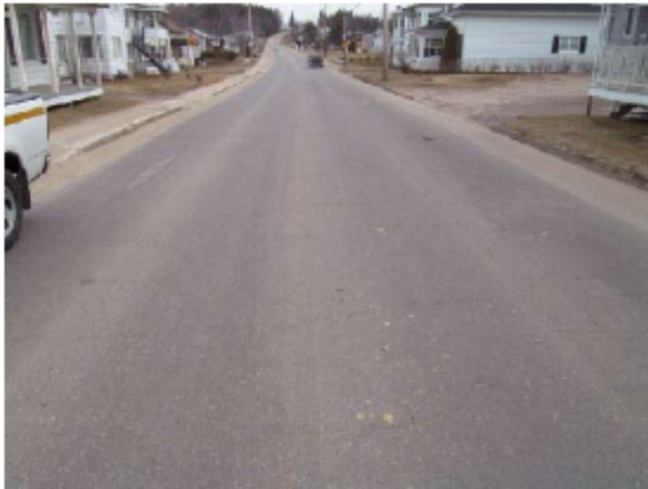
FIGURE 5: Durability Class 5 (85% to 100% Material Loss)
