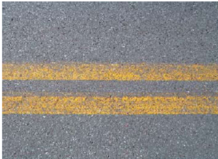
FIGURE 3: Durability Class 3 (50% to 75% Material Loss)
