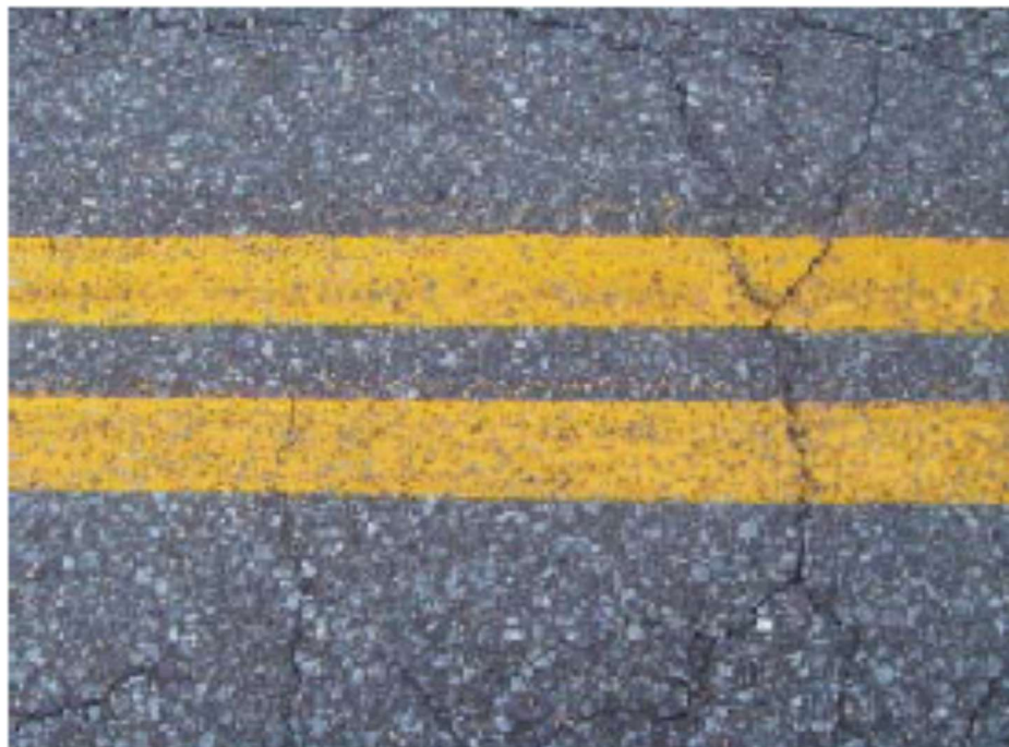
FIGURE 2: Durability Class 2 (5% to 25% Material Loss)
