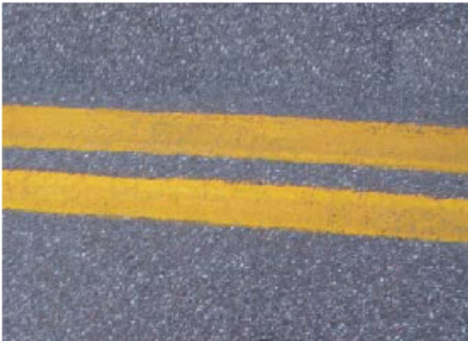
FIGURE 1: Durability Class 1 (<5% Material Loss)
