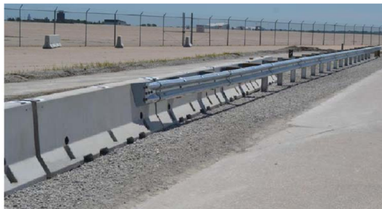
Figure 5- 19 26 : Transition from Existing SBGR to TCB Photo courtesy of MwRSF
