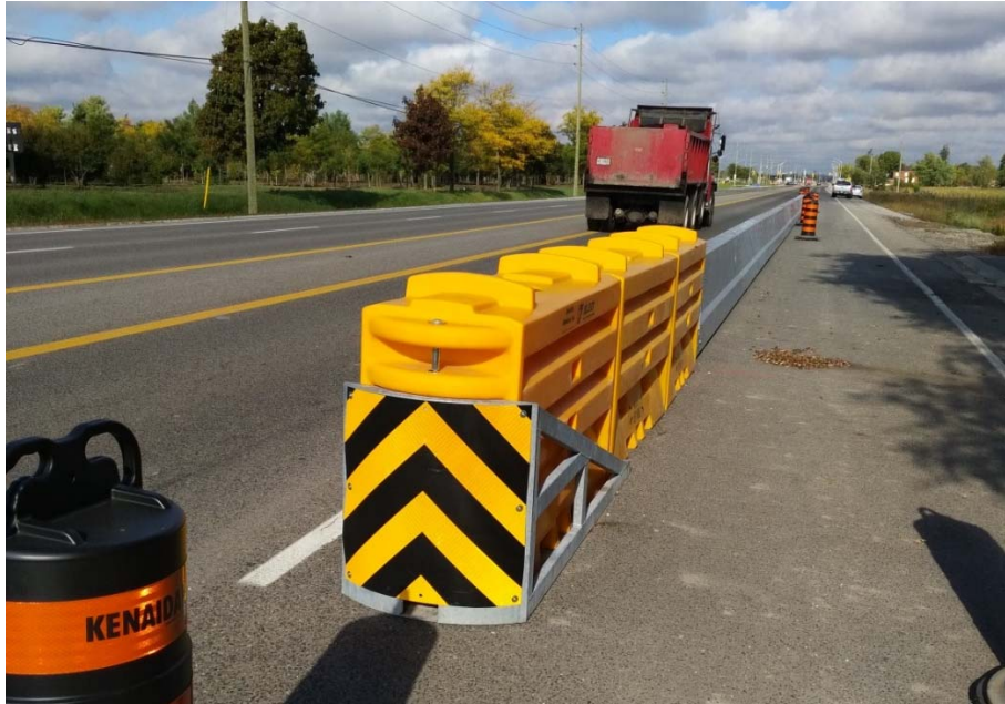
Figure 5- 1825 : SLED Temporary Reduced Exposure Energy Attenuator
