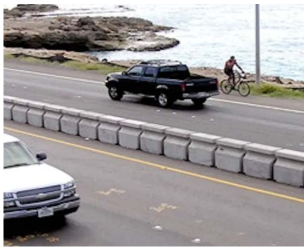
Figure 5-10: Reactive Tension System Barrier Photo Courtesy of Lindsay Transportation
