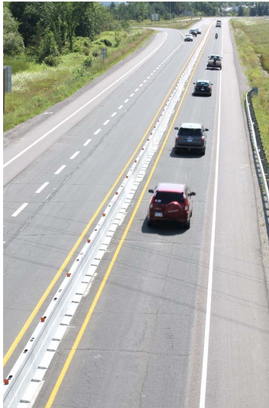
Figure 5-1: Category IV Barrier Separating Staged Opposing Freeway Traffic
