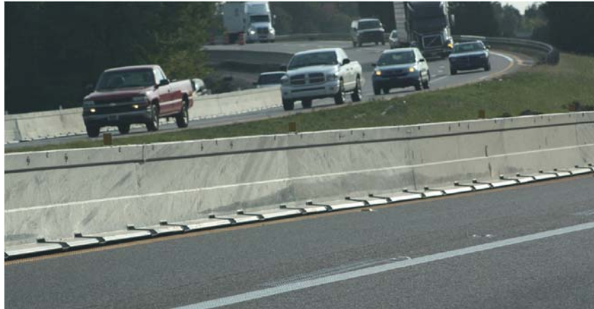
Figure 5-15: ZoneGuard Temporary Steel Barrier Installation
