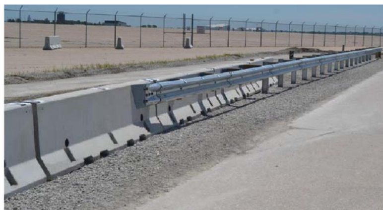
Figure 5-26: Transition from Existing SBGR to TCB Photo courtesy of MwRSF
