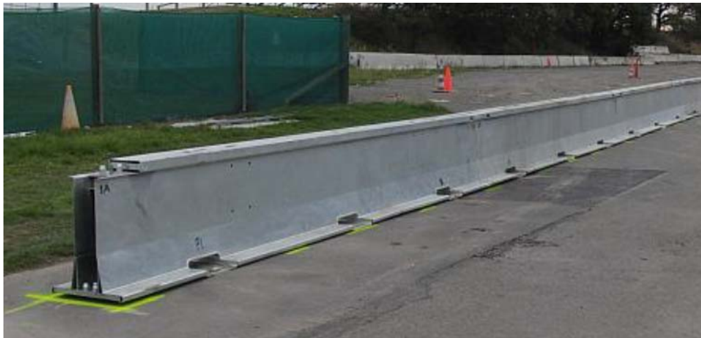
Figure 5-19: Highway Guard Barrier Photo Courtesy of HighwayCare
