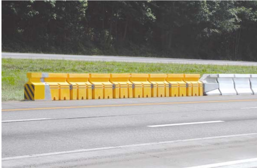
Figure 5-22: Absorb 350 Temporary Reduced Exposure Energy Attenuator
