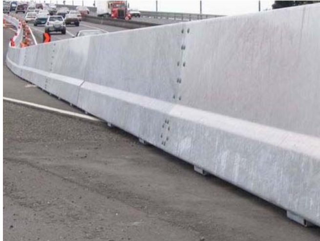
Figure 5-14: BarrierGuard 800 Temporary Steel Barrier
