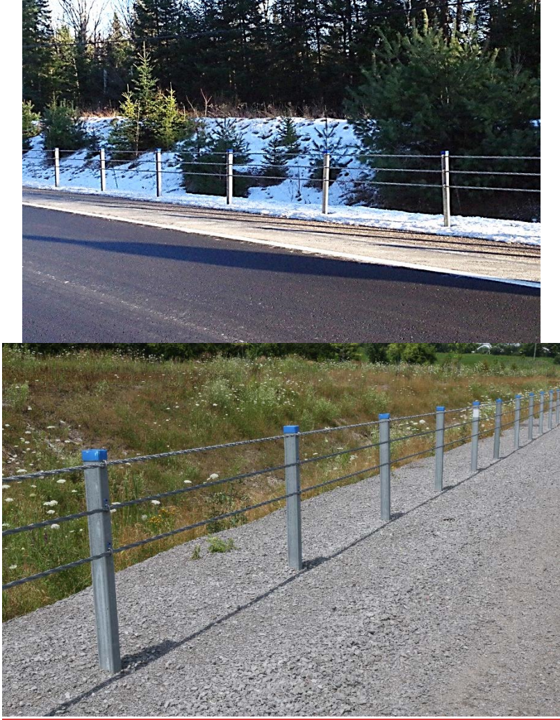
Figure 4-1: Safence HT3CGR Installation
