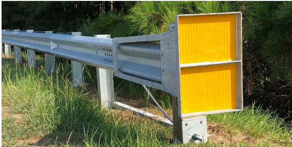
Figure 4-2630: SPIG Gating End Terminal Installation
