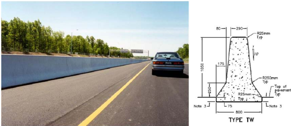
Figure 4- 2023 2024 : Tall Wall Concrete Median Barrier installation
