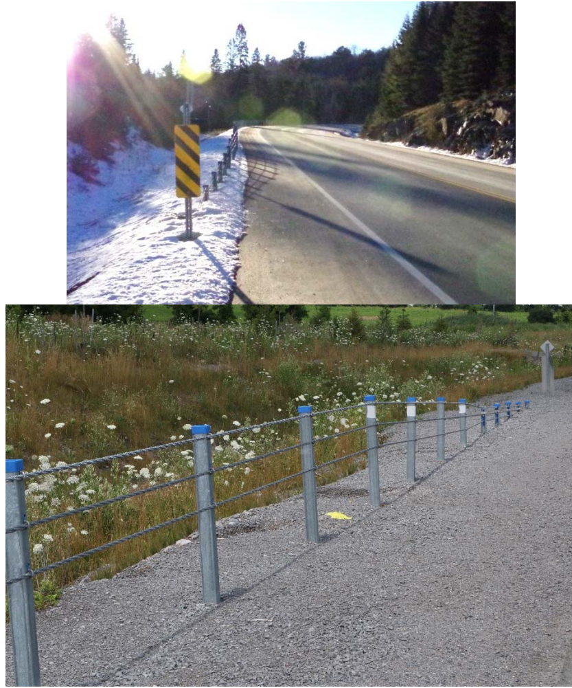
Figure 4-2: Safence HTCGRT installation
