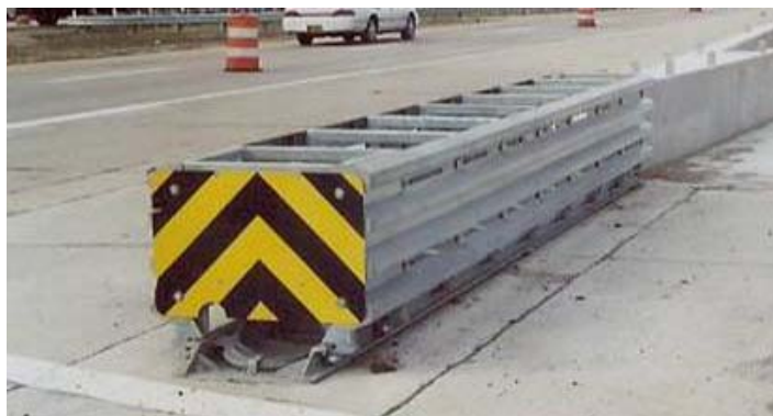
Figure 4- 34 39: SMART Unidirectional Crash Cushion
