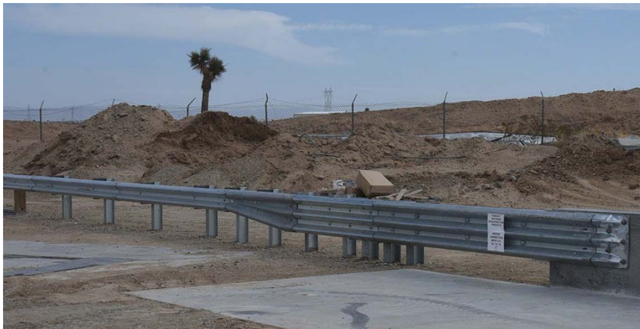
Figure 4-11: MASH Thrie Beam Structure Connection
