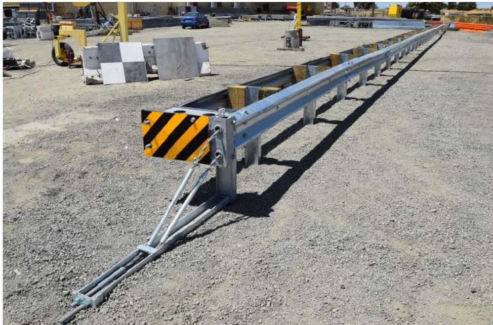
Figure 4-31: Max Tension Median Terminal Installation
