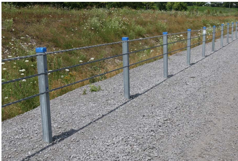
Figure 4-1: Safence HT3CGR Installation
