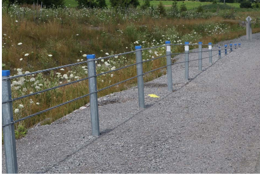
Figure 4-2: Safence HTCGRT installation
