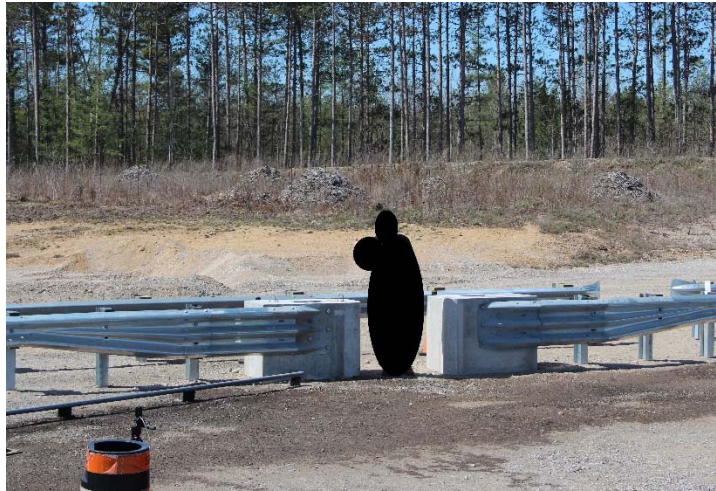
Figure 4-10: Pedestrian Gap for Steel Beam Guide Rail
