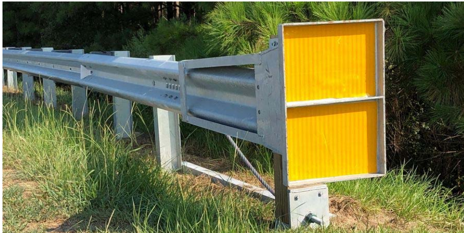
Figure 4-30: SPIG Gating End Terminal Installation
