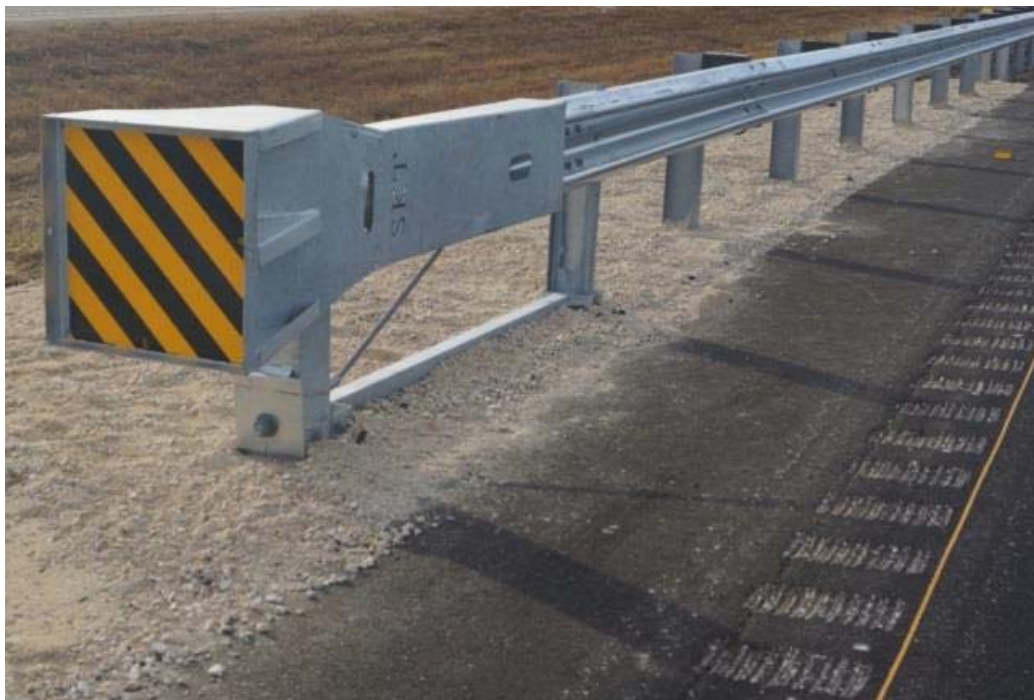
Figure 4-28: MSKT Installation
