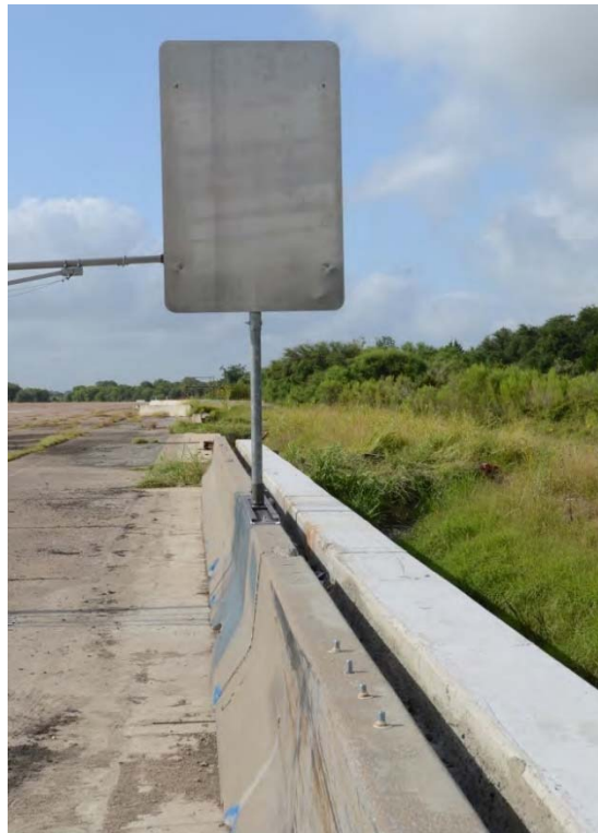
Figure 4-49: Sliding Base and Chute Median Sign Support System Installation
