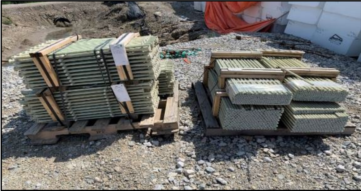
Figure 45 – Good storage cribbing
