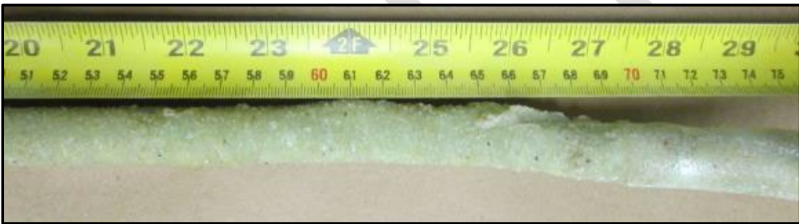
Figure 59 – Out-of-plane bulging larger than 4mm
