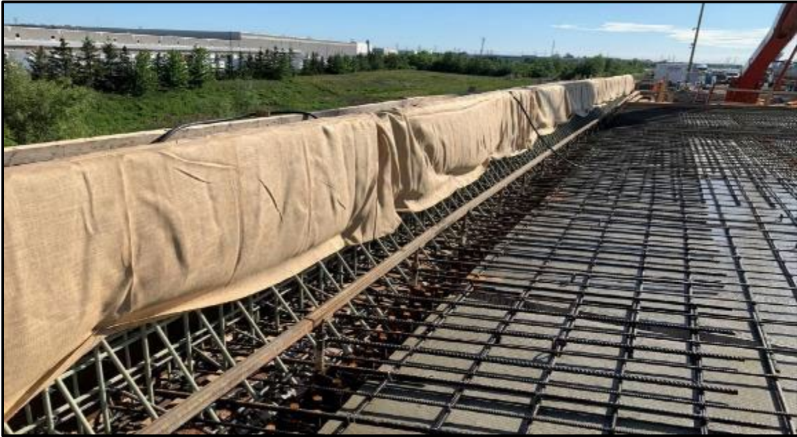
Figure 43 – Barrier GFRP covered with burlap
