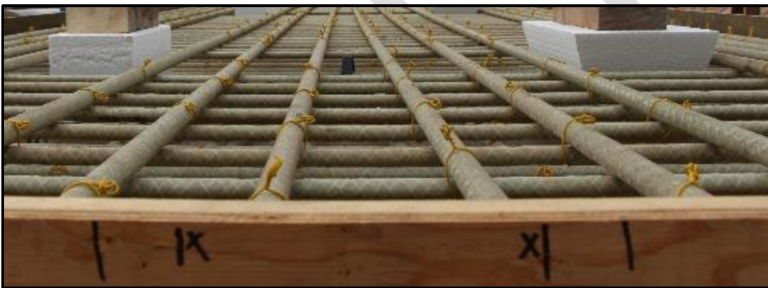
Figure 17 – Straight bars tied in a grid and ready for concrete placement
