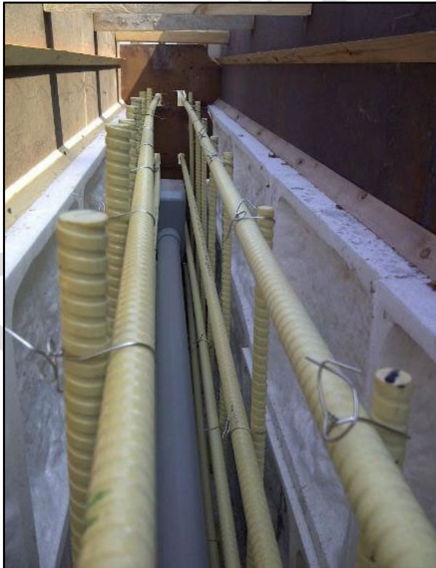
Figure 56 – Acceptable straight bars in formwork (Schöck ComBAR - Fiberline Composites Inc.)
