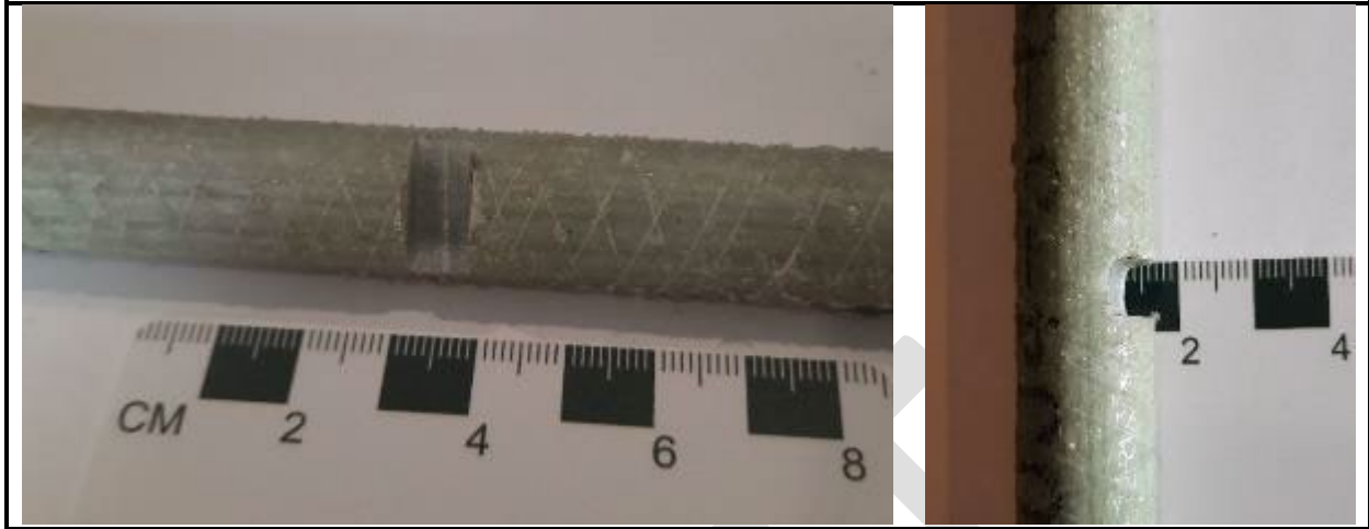
Figure 78 – Deep cut in rejectable bar
