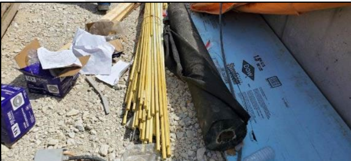
Figure 85 – UV exposure discolouration
