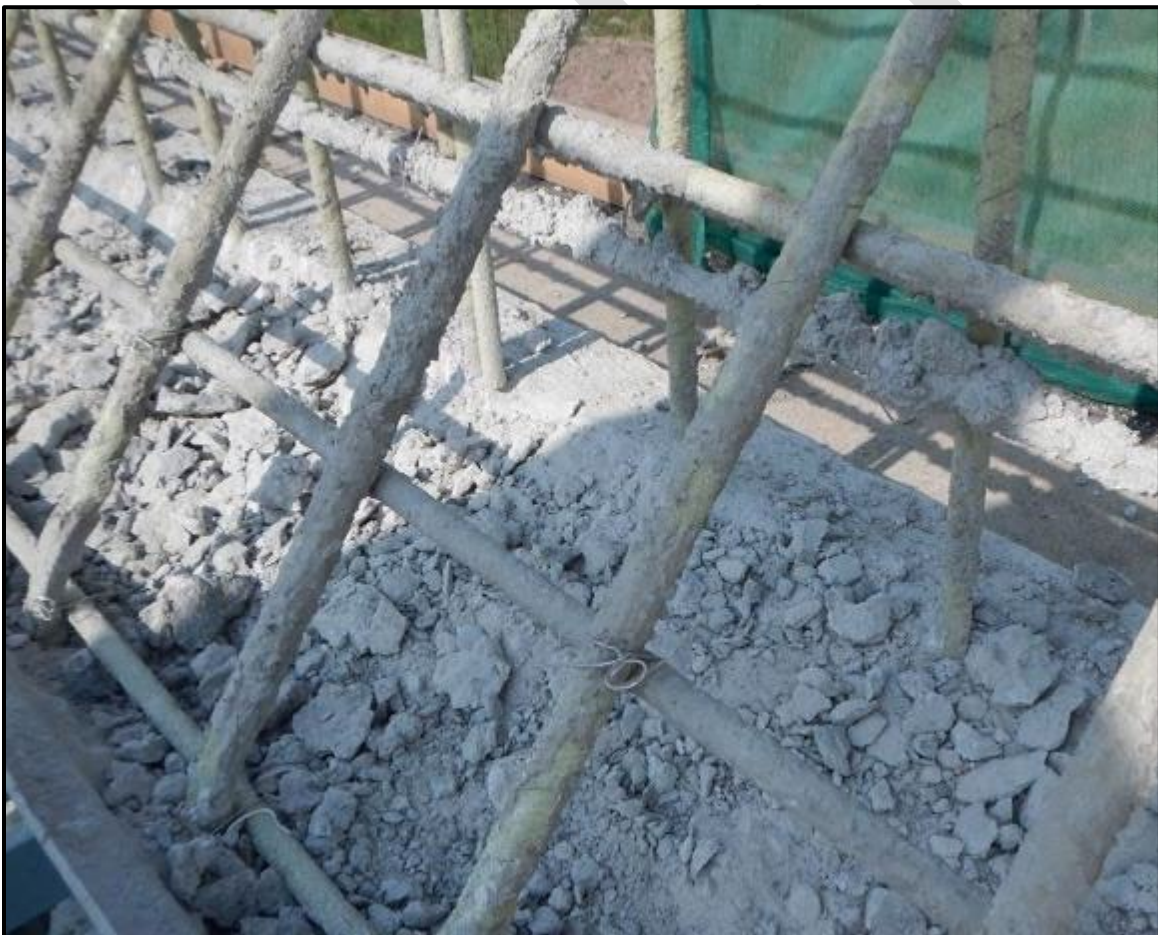
Figure 81 – Concrete contamination
