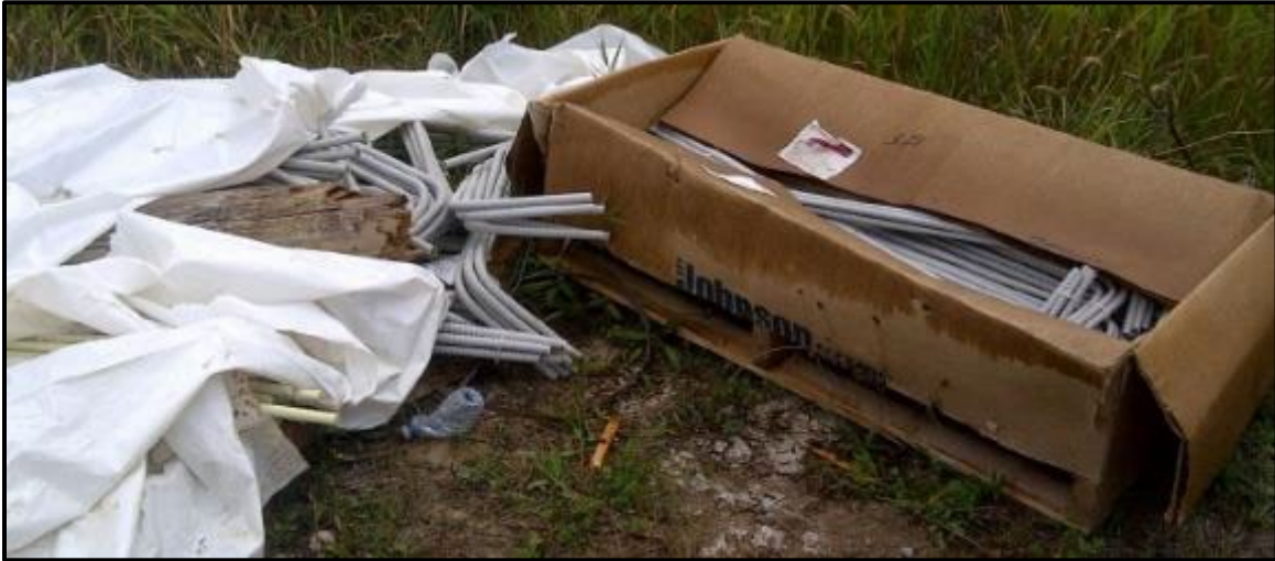
Figure 88 – Not acceptable storage of bars
