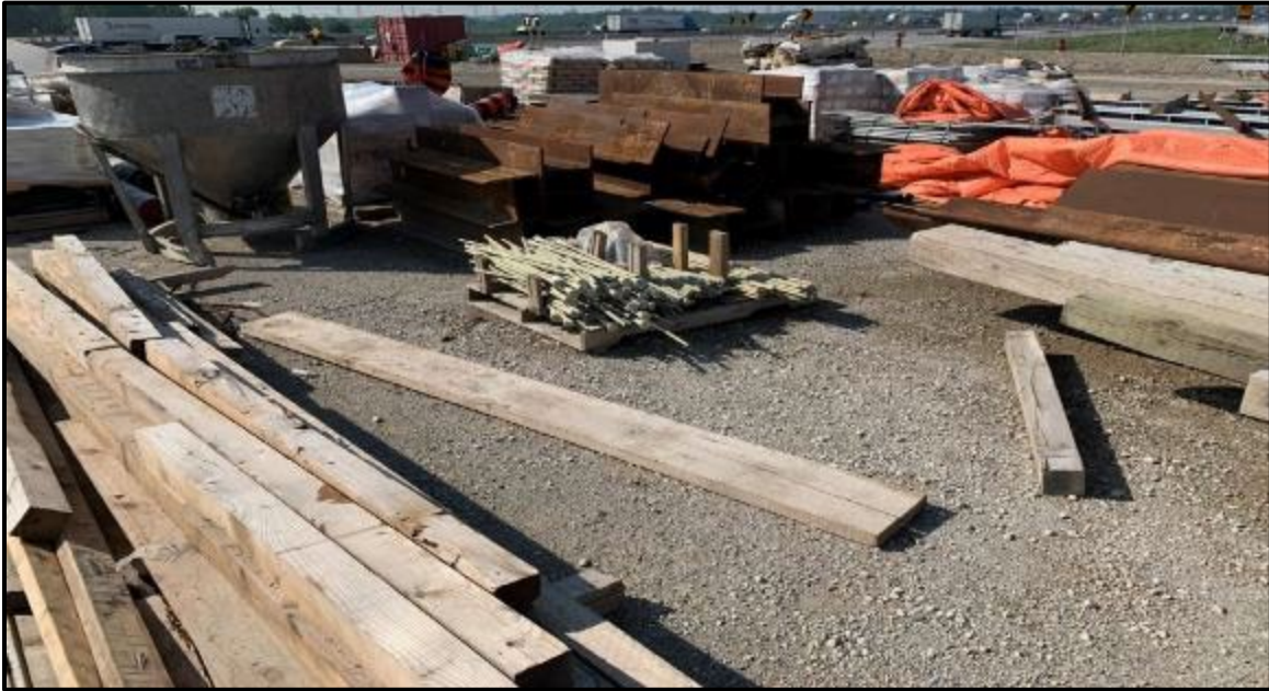
Figure 90 – Bars not covered with polyethylene
