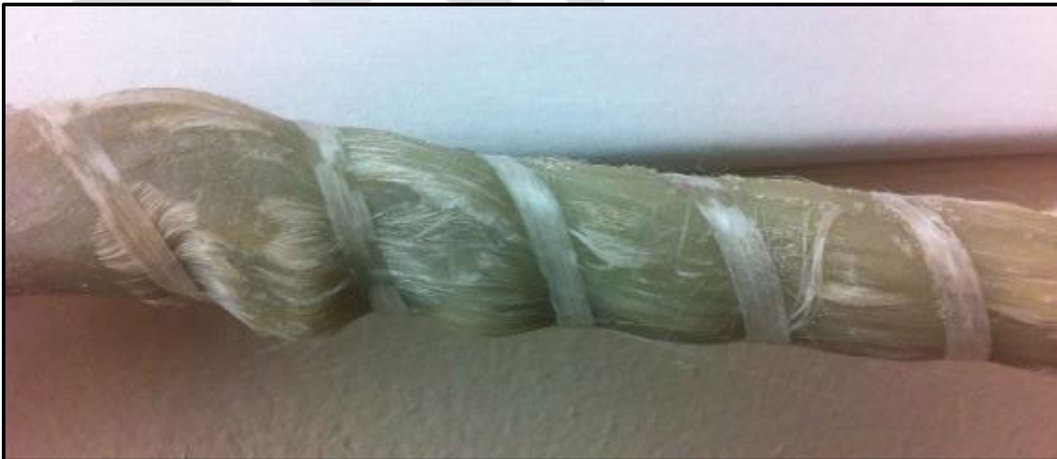
Figure 60 – Bulging fibres and inconsistent resin coating
