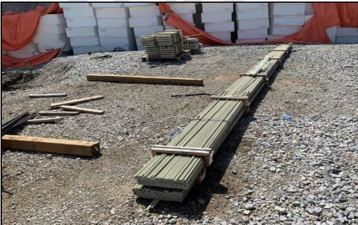
Figure 89 – Bars not covered with polyethylene
