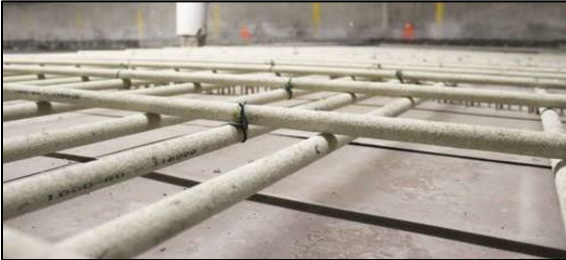
Figure 16 – Straight bars tied in a grid and ready for concrete placement
