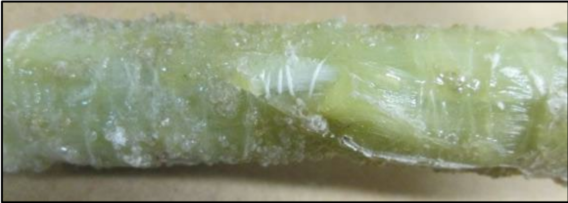
Figure 67 – Repairable exposed fibres
